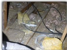
Some of the insulation has been disturbed. It is recommended that the insulation be redistributed, and improved as necessary to ensure consistent comfort levels throughout the home.
