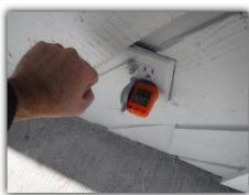
Exterior receptacles are currently required to have a "weatherproof while in use" cover, also known as a plastic "bubble cover" type.
