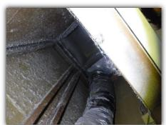
The return filters are missing or dirty. Missing or dirty clogged filters make the unit work harder and cuts down on the efficiency and life of the unit.
