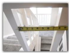
■ Space between railings does not comply with current industry standard, Requires spacing between intermediate rails do not allow passage of an object four inches in diameter.
