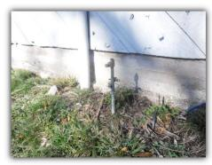
The main electrical service grounding electrode was not visible at the time of the inspection. A grounding electrode conductor was visible exiting the main panel and entering soil, but the inspector was unable to confirm its proper termination or proper grounding of the electrical service. Although this is a common condition, you may wish to have proper grounding conditions confirmed by a qualified electrical contractor for safety reasons.
