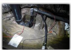
Air-conditioning refrigerant and drain lines should be checked, insulated, and cleared as necessary
