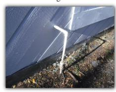
Note: The visible portions of the water pipes in the attic are not insulated. Recommend insulating exterior water line(s) to prevent freeze damage.
