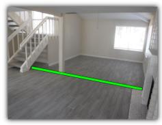
Tripping hazard, there is no contrasting color at raised section of flooring;
