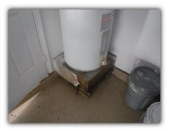
Note: Manufacturers recommend flushing and draining a water heater annually to remove sediment that accumulates on the tank bottom. This procedure involves connecting a hose to the drain valve at the bottom of the tank, and allowing the water to flow until it appears to be clear. Problems that may arise from sediment accumulation include reduced heat exchanger life on gas-fired models, and premature lower element failure on electric models.
