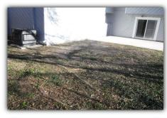
■ The drainage and grading around this home is inadequate. In order for the drainage to be effective, the landscaping must be configured so that the yard is sloped away from the foundation by at least 6 inches in the first 10 feet and/or adding additional gutters/downspouts to the house is another option to improve drainage and/or in- ground drains should be designed and added to divert rainwater and runoff away from the house as appropriate and/or drainage swale should be improved/installed.
