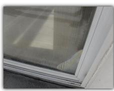
Thermal pane window on sliding door seals have failed, and moisture has penetrated.
