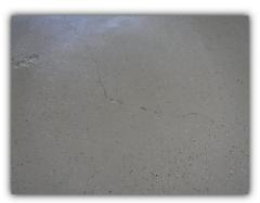
Cracks in a concrete garage floor. Most cracks in garage floors are common and not an indication of serious structural issues, however there are a few that indicate that maintenance is needed or that there may be a structural concern.
