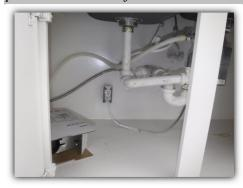
■ The drain line was not raised as high as possible, and secured under the cabinet in order to help prevent possible back-siphoning at the time of the inspection.
