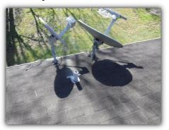
Satellite dishes are not recommended to be mounted on the roof covering. The mounting process may for water intrusion
