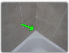
☐ The tub enclosure needs to be sealed. Grout / caulking needed at vertical tile corners, cracks in tile and/or mortar between tiles, and where tile meets tub to prevent water entry behind wall.
