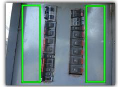
All fuse or breaker panels are required to have an complete, legible, and accurate listing of what the circuits are connected to. This is properly called a legend.
