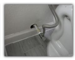
Observed deficient flushing mechanisms. Replacing the commode's flushing mechanisms supply hoses as a and water preventative measure before occupying the house is recommended.
