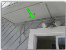
Missing light fixture / exposed wires were noted.
