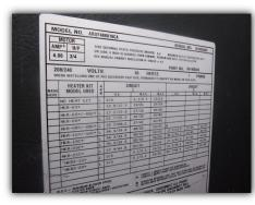
The photo shows the furnace make, model and serial numbers marked on the furnace label or data plate.
