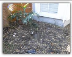
The grade around the house should not have any low-lying areas but should be sloped so that water will not collect and puddle here and there.
