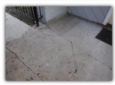
The walkway is cracked and appears to have some movement in the elevation of the concrete. The elevation differences can be a trip hazard as well as contribute to the deterioration of the driveway. I recommend having a qualified contractor evaluate and repair as needed.
