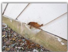
Water damaged was noted in wood siding at one or more location and it is recommended that the damaged wood be repair and/or replaced.
