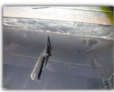
The normal use of a fireplace can result in excessive build up of creosote or a tar like substance. Chimney flue should be cleaned and/or serviced on a regular basis or as specified by the manufacture.
