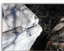
Mortar cap needs repair at top of chimney, if visible
