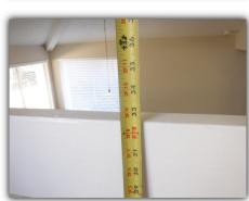
■ The hand railing is not at the proper height, which is 34-38 inches high. The hand railing was measured at 33.inches at the time of the inspection.
