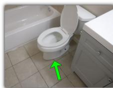
The floor mounting is loose. The commode(s) needs to be sealed/caulked.
