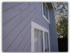
The window and/or door and/or other wall penetrations installed through the wood fiber products siding were not properly flashed.
