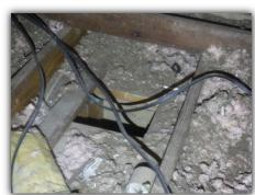
There were areas that appear to be open between the attic floor and ceiling below. The chase should be covered with a fireproof material, then insulated.
