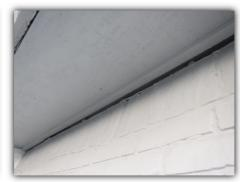
Gaps should be sealed from rodents, also may allow wind driven rain entry. Recommend sealing all gaps to keep the house from rodent and water intrusion.
