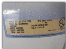
The photo shows the water heater make, model and serial numbers marked on the unit label or data plate.
