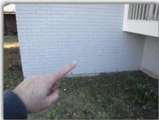
A stair-step crack is a diagonal, right-angle crack that travels through the mortar surrounding the brick since mortar is not as strong as brick. The resulting crack looks like a staircase going up and down. A stair-step crack will usually point to the area of the foundation that is sinking or settling.
