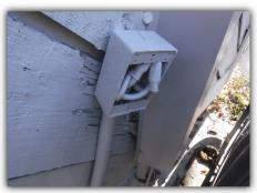
Service disconnect for the air conditioner is missing. Recommend installing electrical disconnect within sight of unit.
