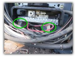
There is double lugging of the neutral wiring in the service panel. Each neutral service wire is required to be under one screw per wire.
