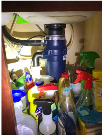
General Photos of Range Hood/Exhaust Systems:
