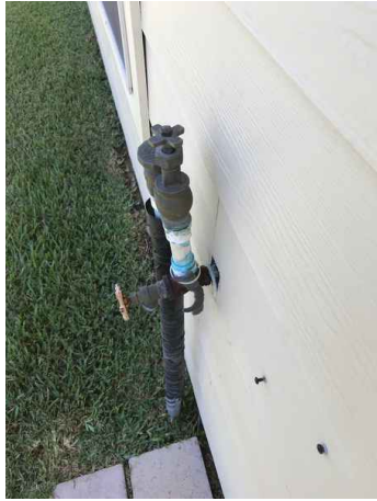
Filtering Components:: Pool Sweep, Skimmer
