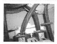
There were "white wires" attached to breakers. White wires are deemed neutral and must be identified as bot wires by tape or red or black paint at breaker end.
