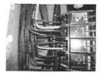
Most of the supply wires are bundled where they go out of the main panel, this is common on most older homes but is not proper per current electrical standards.
