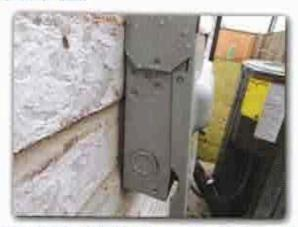
The exterior outlets are weather sealed but not caulked,
