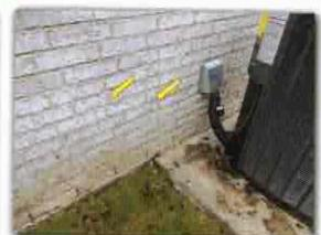
The A/C emergency shut off switch boxes are not properly weather sealed/caulked at the exterior wall.
