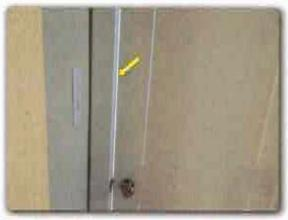
There is daylight showing through the backyard door jamb. This is indicative that the door is not fully weather sealed.
