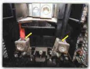
The bonding screw is not installed in the main panel. This is required to ensure that the neutral bar is secured to the panel. I was able to locate it sitting at the bottom of the panel. This needs to be installed.
