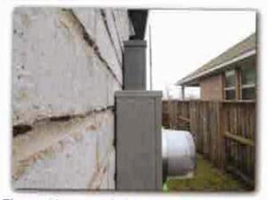
The vent is not sealed to the wall.
