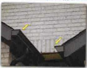
The flashing needs to be sealed on the front right side.
