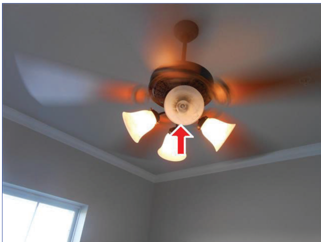
B. Item 1(Picture) This light failed to light with activation of the light switch.
