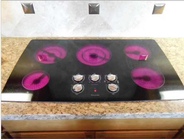
D. Item 3(Picture) View of the cooktop functioning.
