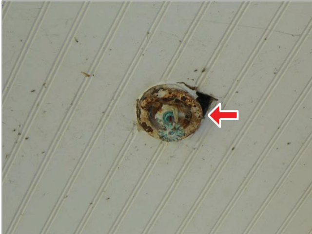
L. Item 1(Picture) Excessive rusting of fire suppression sprinkler
