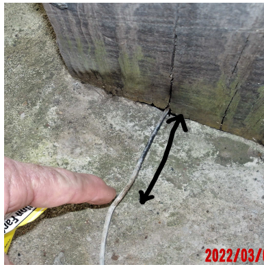
Piling erosion.
