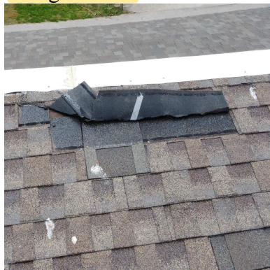
Damaged roofing.
