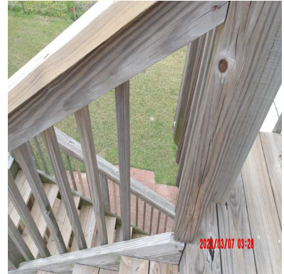
Missing baluster.
