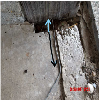
Piling erosion.
