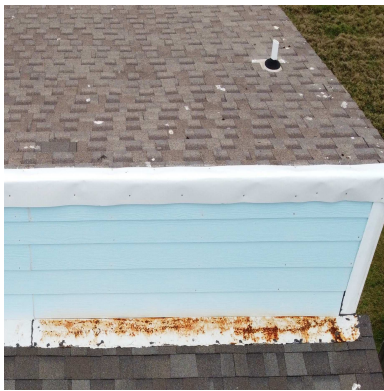
Rusting flashing.
