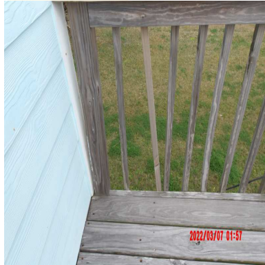
Broken baluster.
