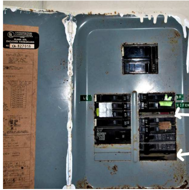
Missing knockouts.
