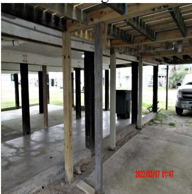
Temporary bracing under the deck.
