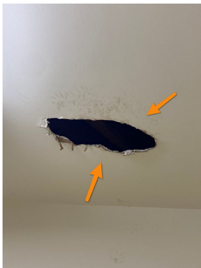
2nd Floor Closet
