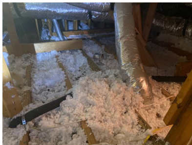
Viewed From: Attic
