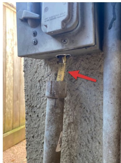
Under breaker box
