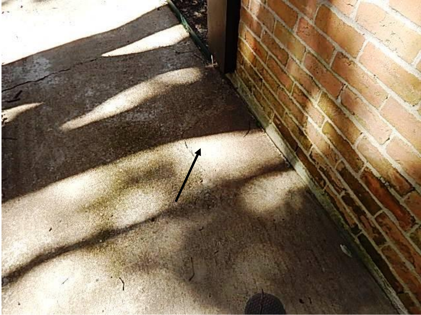
Evidence of prior pier installs.
