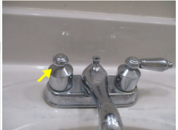
Broken handle at hot side of left sink fixture in addition bathroom.
