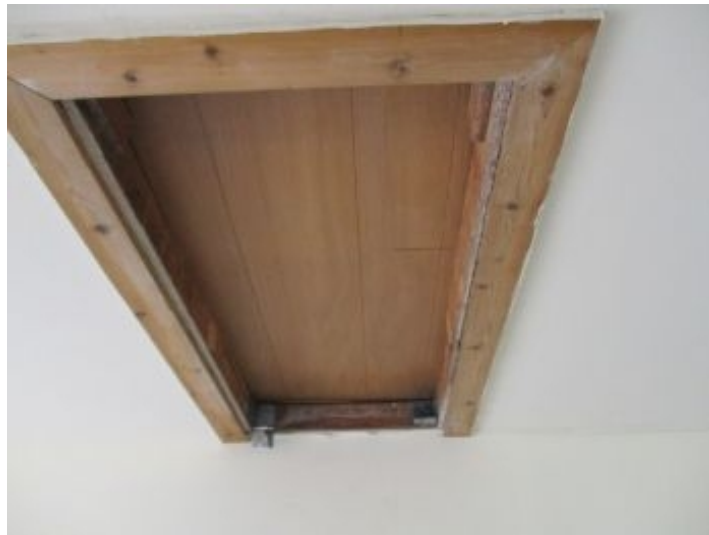
Pull down attic stairs have been removed.
