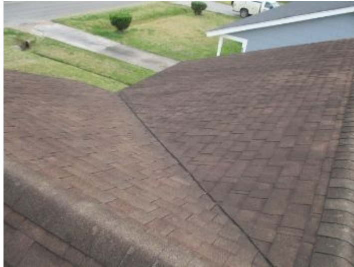
A view of roof
