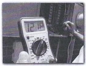
200amp service panel-150amp main- 120/240v copper wired breaker service. Breaker wiring, buss bar shields and breakers showed no indications of over heating or arcing and were observed to be in good condition at this time.
