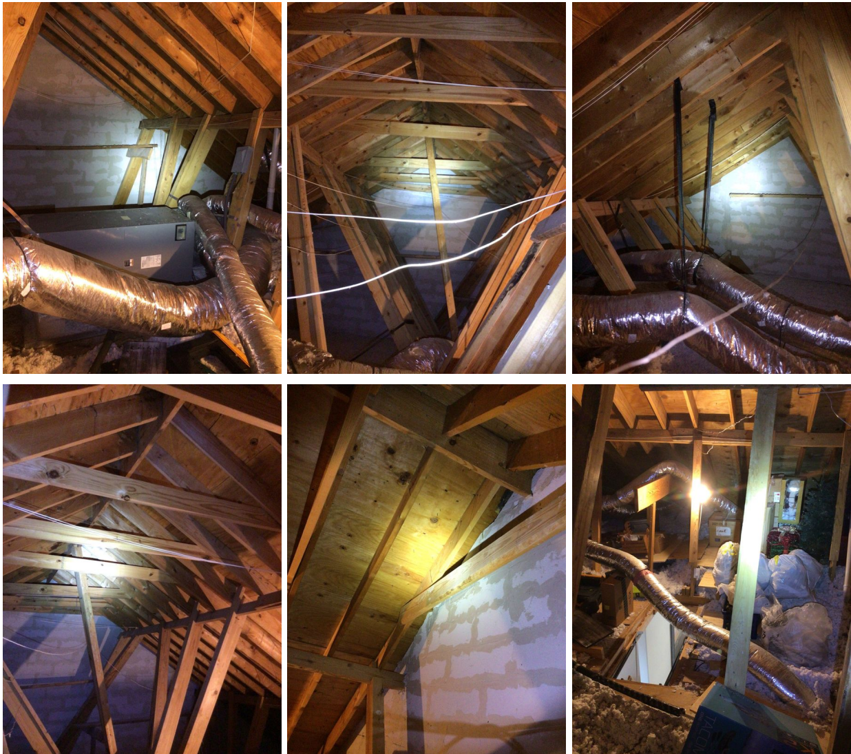
General Photos of Roof Covering:
