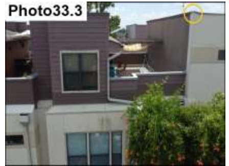
Metal Cap/Siding Termination / Seal
