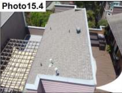
Roof Flashing / Seal
