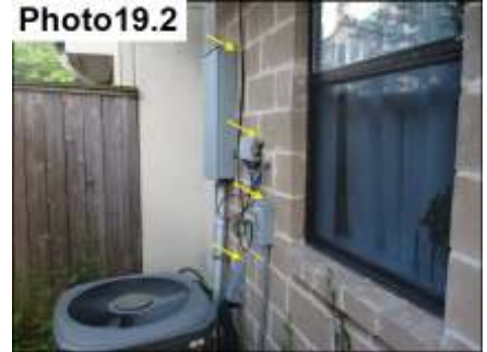
Penetration Sealants / Seal
