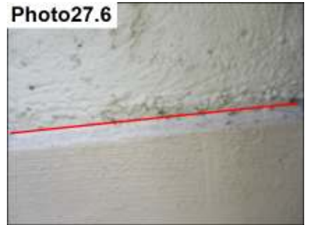
Window Accent Band/Stucco Termination / Seal
