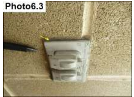
Penetration Sealants / Seal
