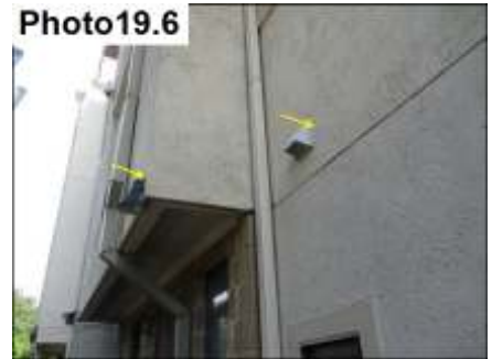
Penetration Sealants / Seal
