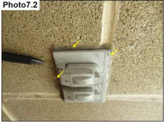
Penetration Sealants / Seal
