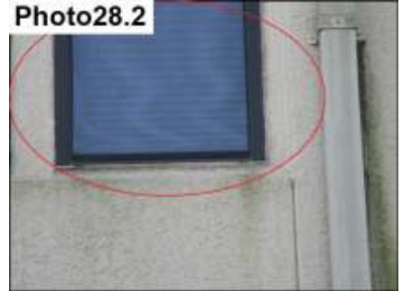
Refasten & Seal All Screws Then Wet Glaze
