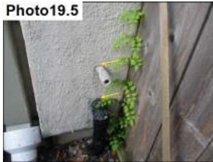
Penetration Sealants / Seal
