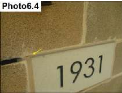
Penetration Sealants / Seal
