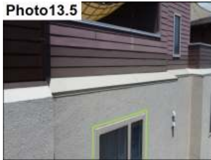
Window Accent/Stucco Termination / Seal
