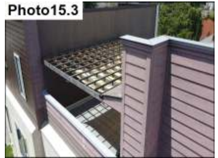
Roof Flashing / Seal
