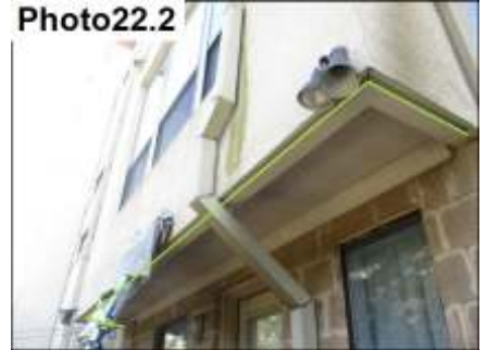
Reglet Vent Installed / No Modification
