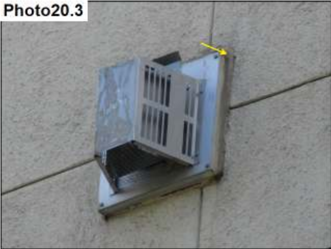
Penetration Sealants / Seal
