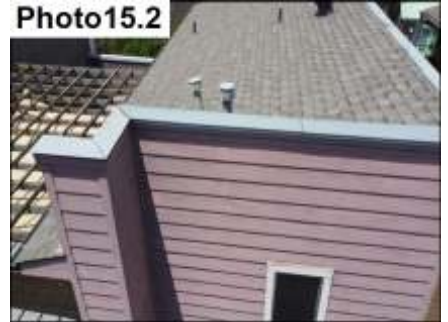
Roof Flashing / Seal
