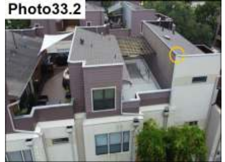
Metal Cap/Siding Termination / Seal
