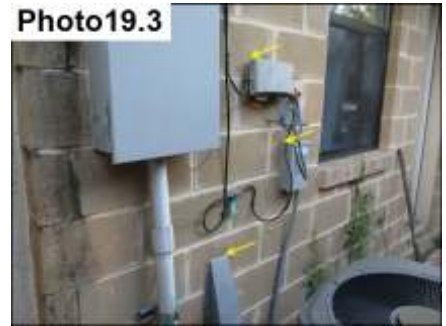
Penetration Sealants / Seal
