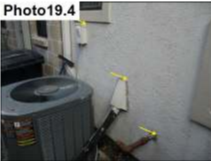
Penetration Sealants / Seal
