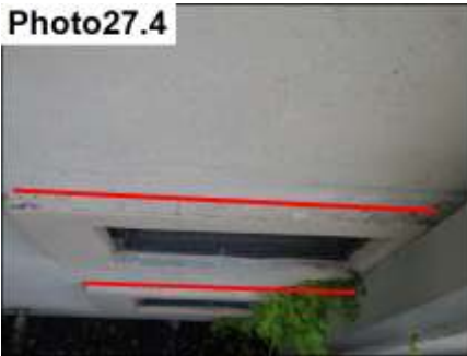
Window Accent Band/Stucco Termination / Seal
