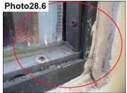
Refasten & Seal All Screws Then Wet Glaze
