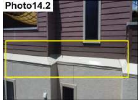
Metal Cap/Siding Termination / Maintain
