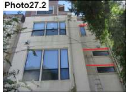
Window Accent Band/Stucco Termination / Seal
