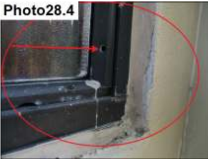
Refasten & Seal All Screws Then Wet Glaze
