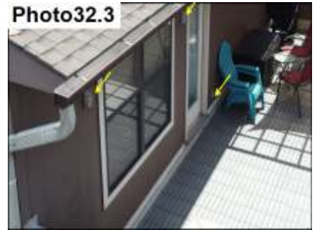
Penetration Sealants / Seal
