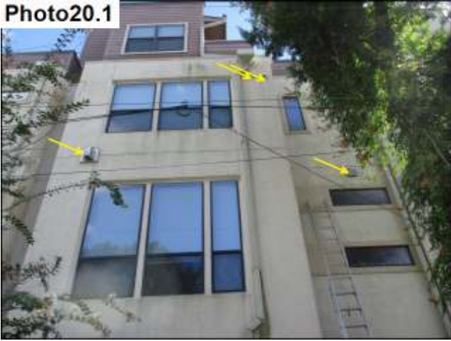
Penetration Sealants / Seal
