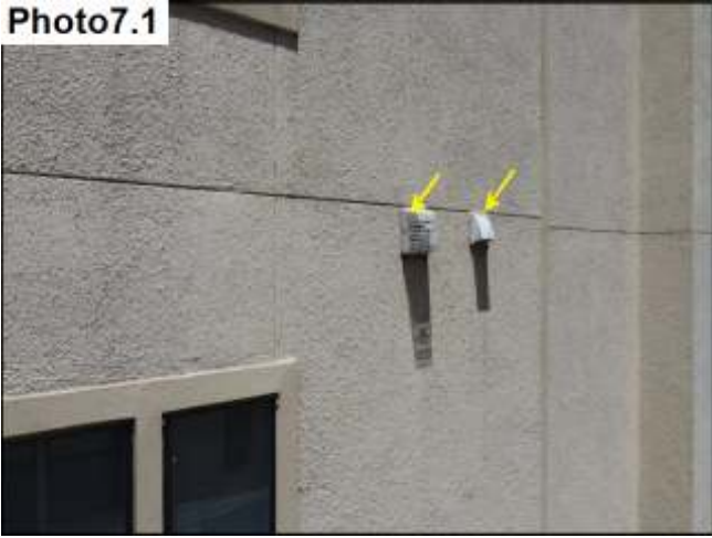
Penetration Sealants / Seal
