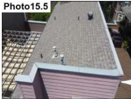
Roof Flashing / Seal
