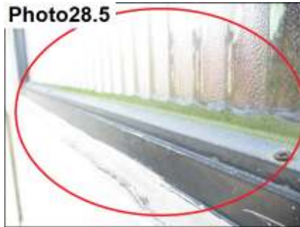
Refasten & Seal All Screws Then Wet Glaze
