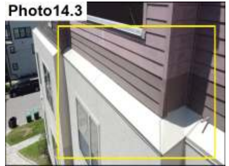
Metal Cap/Siding Termination / Maintain
