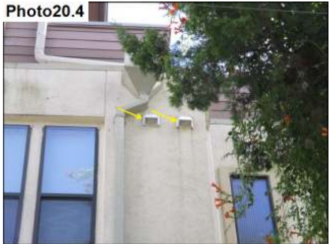
Penetration Sealants / Seal
