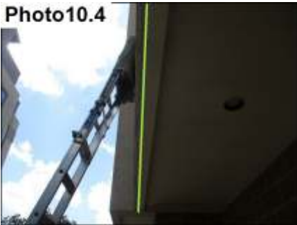
Reglet Vent Installed / No Modification
