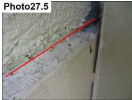
Window Accent Band/Stucco Termination / Seal
