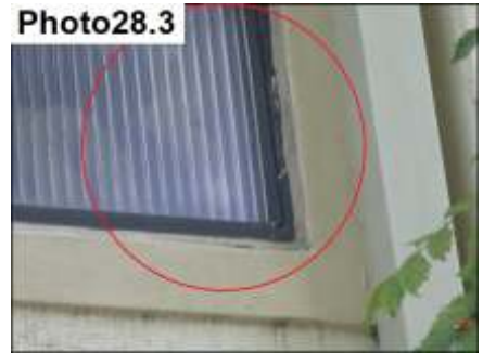
Refasten & Seal All Screws Then Wet Glaze
