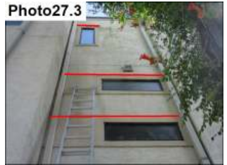
Window Accent Band/Stucco Termination / Seal
