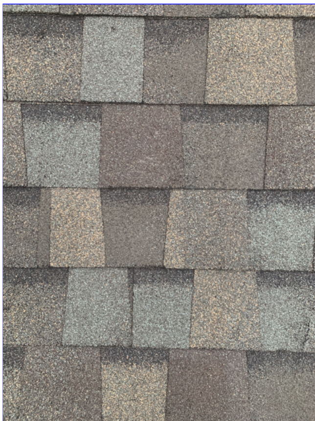
C. Photo 1(Picture) This roof is an Architectural style shingle that will typically last 20 years in this climate.
