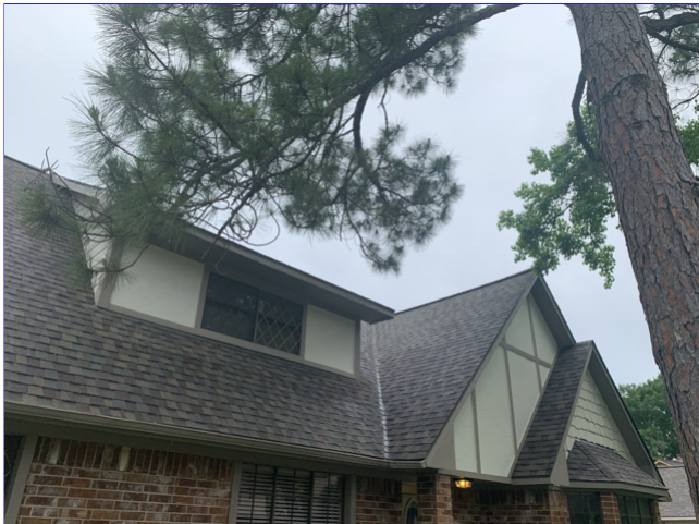
C. Photo 2(Picture) Note: Tree limbs that are in contact with roof or hanging near roof should be trimmed. Tree limbs in contact with the shingles can cause damage.
