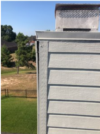
The trim board on the chimney is split and warped away from the chimney. Recommend a licensed professional repair the trim. The cabinet to the right of the dishwasher is pulling away from the wall at the top and needs to be secured.
