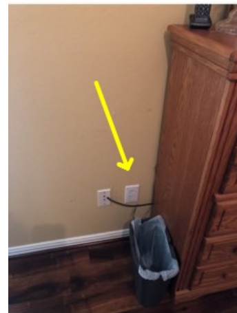
(Informational) The receptacle on the right wall of the middle bedroom is loose.
