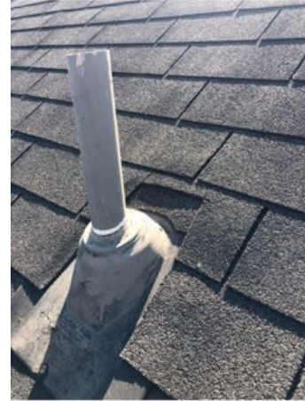
Shingles are lifting at the top of the roof jack..
