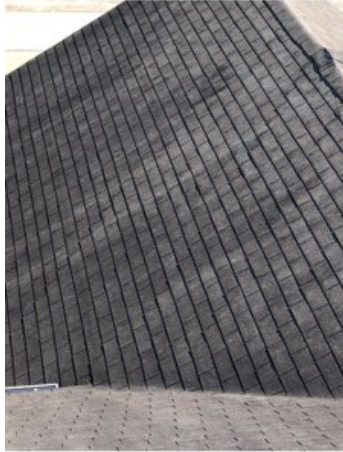
The shingles are starting to lift and come loose. The shingles are nearing the end of their life cycle.
