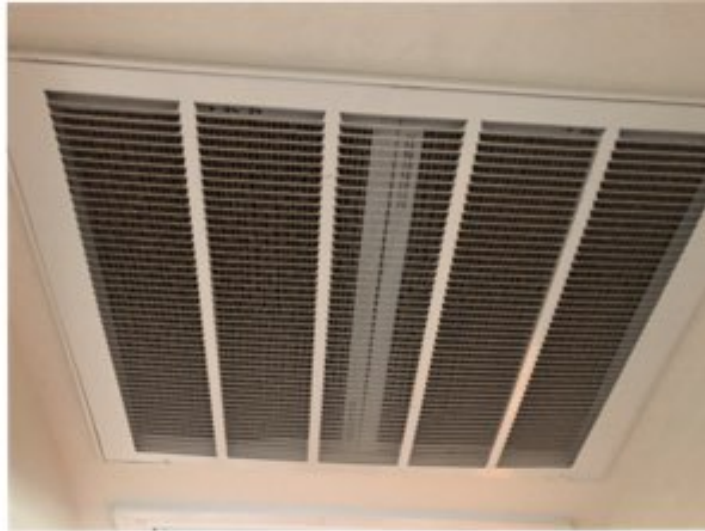
The return air register and the filter is dirty. There are two filters 10 X 25 X 1.
