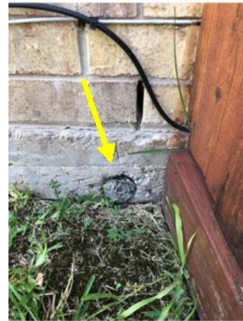
Cable ports on post tension foundations should be sealed with mortar.
