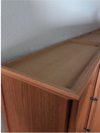
The cabinet to the right of the dishwasher is pulling away from the wall at the top and needs to be secured.
