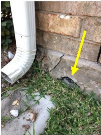
Cable ports on post tension foundations should be sealed with mortar.
