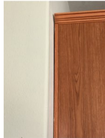
The trim board on the chimney is split and warped away from the chimney. Recommend a licensed professional repair the trim. The cabinet to the right of the dishwasher is pulling away from the wall at the top and needs to be secured.
