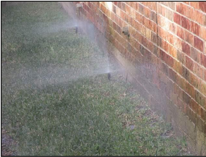
30. Sprinkler heads should be adjusted to spray...
