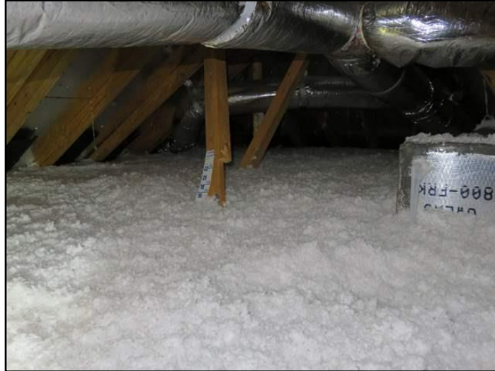
14. General view of attic insulation.
