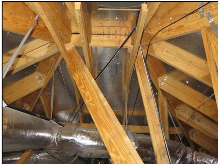
7. General view of attic structure.
