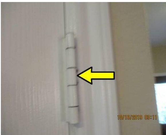
Door leading to the garage should have self closing hinges
