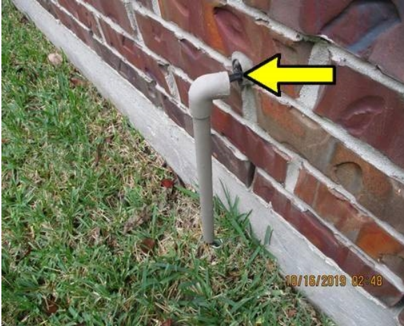
Seal around penetrations (Irrigation wire)
