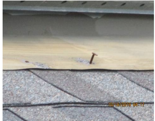
Secure and seal flashing nail above front porch
