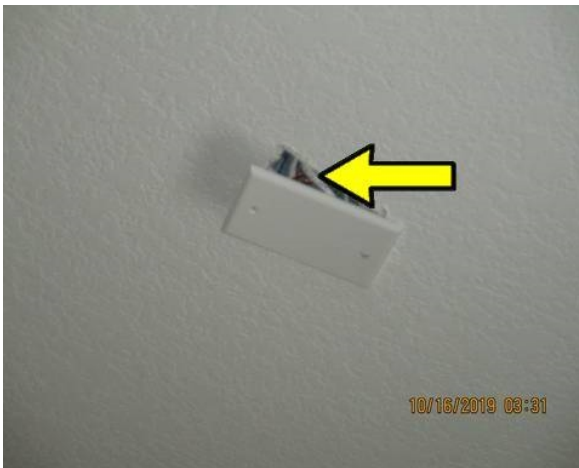
Secure speaker wires in ceiling at upstairs game room
