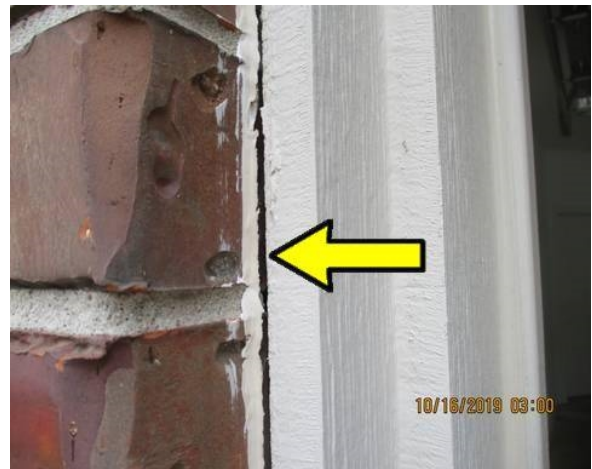
Repair caulk around overhead garage door frame
