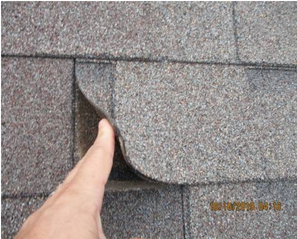
Shingles are still pliable
