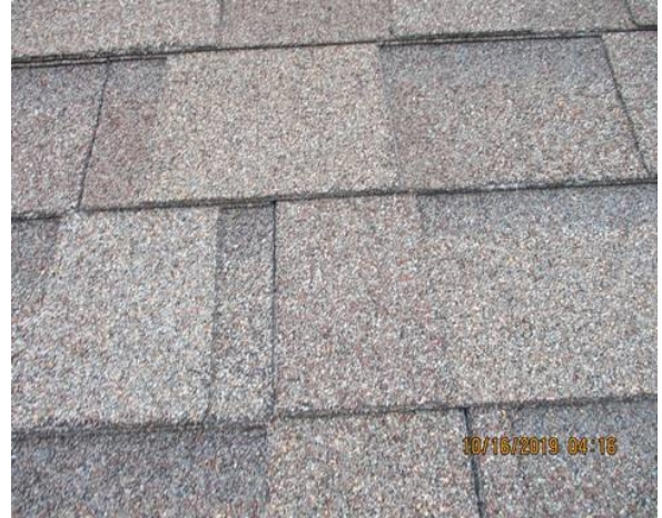
Condition of shingles
