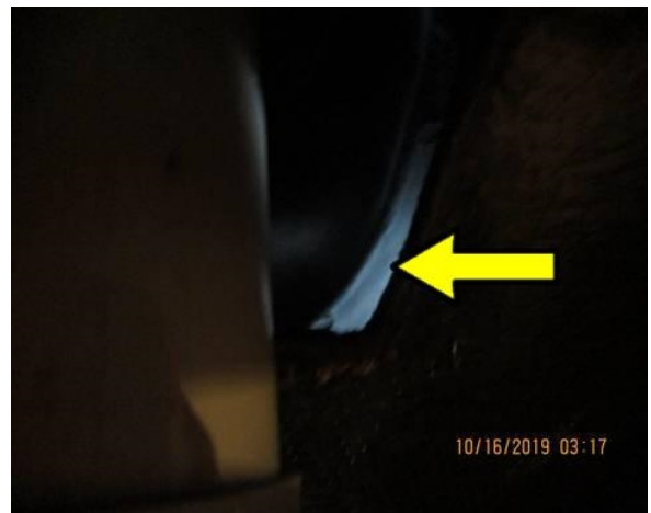
Outside light is visible around furnace flue vent
