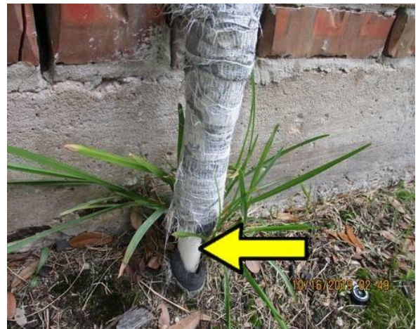
Repair insulation on water main shut off
