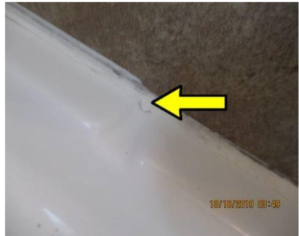
Remove caulk around weep holes at master shower pan
