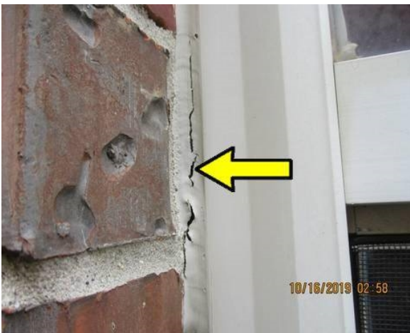
Repair caulk around windows
