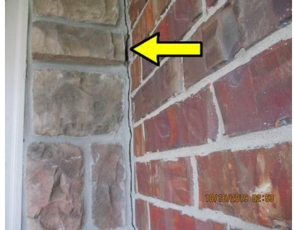
Seal mortar at right of front door
