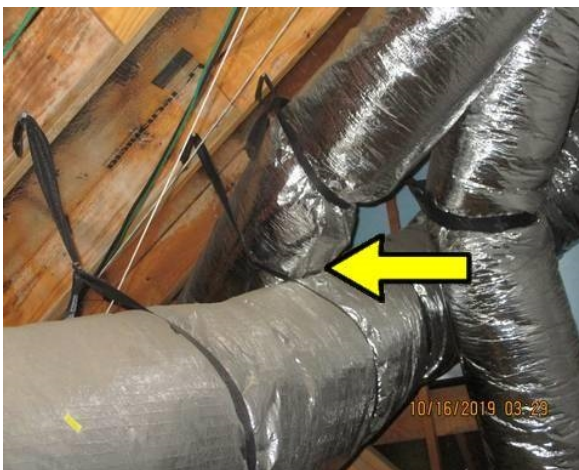
Add batt insulation between ducts that touch
