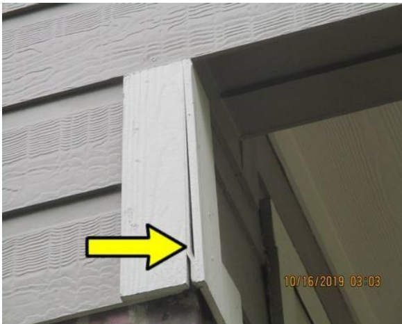
Secure and seal trim piece at back patio
