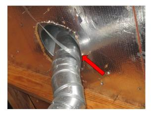
The gas line for the heating system is in contact with the heating vent. There should be a minimum of 1 inch clearance to all combustible materials.
