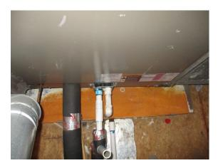
There is what appears to be a fungal growth on the evaporator coils and plenum in the attic. Recommend further evaluation and repairs by a licensed HVAC contractor.
