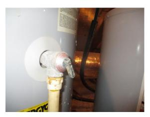
The water heaters make a popping sound when the water is being heated. This usually indicates a layer of sediment in the bottom of the tank and makes the water heater less fuel efficient and recovery times longer. Recommend further evaluation by a licensed plumber.
