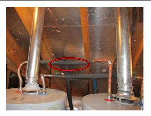
The floor under the water heaters in the attic appears to be bowed. Recommend further evaluation and repairs to ensure the water heaters are properly supported.
