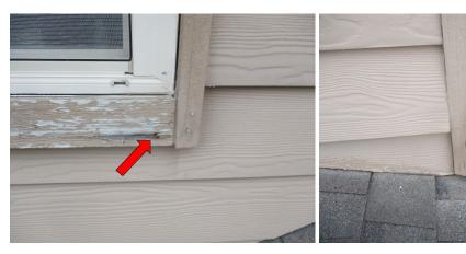
There are gaps between the baseboards and where the baseboards and walls meet. Recommend caulking.
