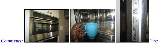
10/2015 "*General Electric*" Microwave oven performed as intended on the day of the inspection. It heated a cup of water to steaming after one minute of operation.
