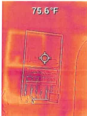
Some conditioned air loss from the windows
