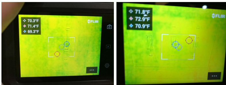
General Photos of 220V Outlets:
