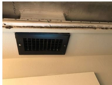
1st Floor Bathroom
