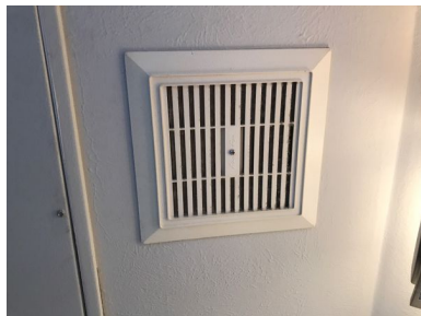
1st Floor Bathroom
