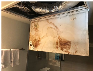
2nd Floor Bathroom
