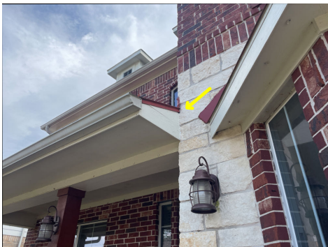
Improper flashing.
