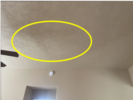
Repair to ceiling.
