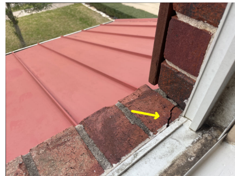
Brick crack.
