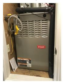
1: Gas Piping: Missing or Improper Drip Leg
