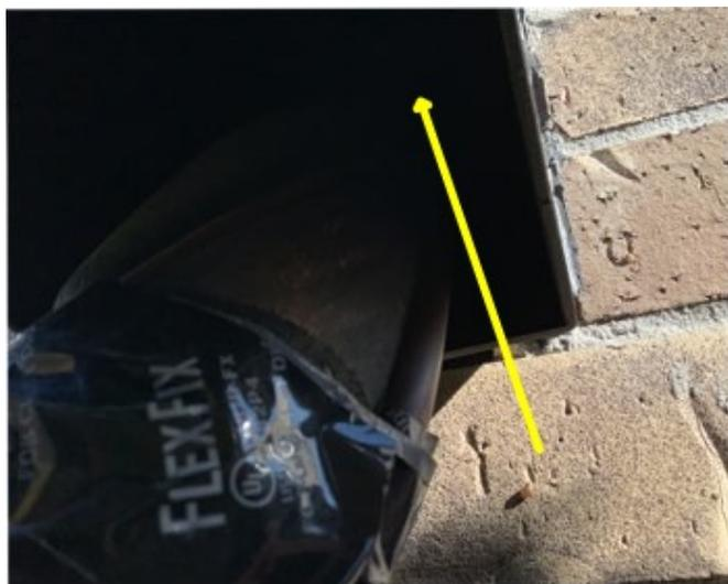
Under the shroud where the refrigerant lines enter the dwelling needs to be sealed to prevent rodents and insects from entering.
