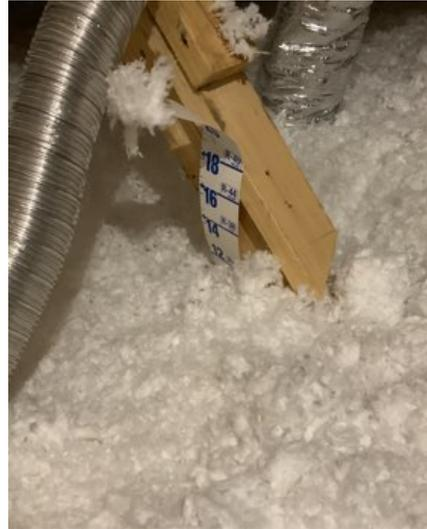
12 inches of blown in fiberglass present in downstairs attic
