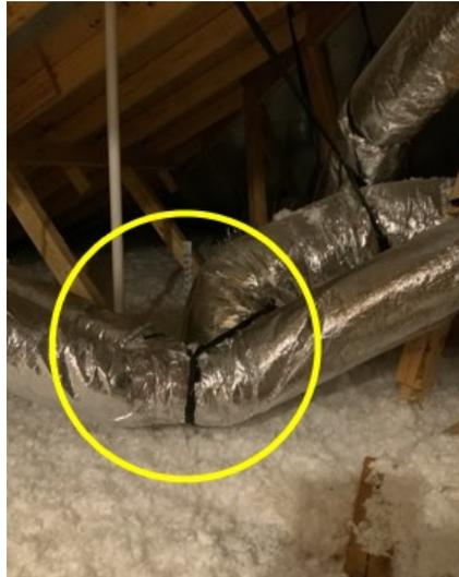
The duct strapping broke causing the ductwork to collapse above primary bedroom
