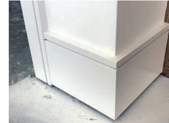
Baseboard & Door/Window Casing
