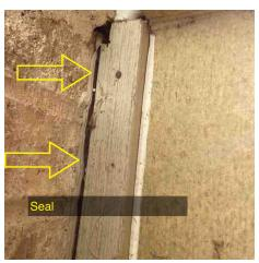
• Seal gap in brick to prevent moisture intrusion.
