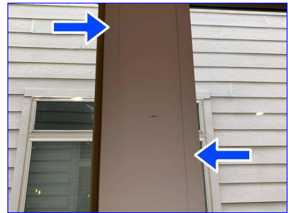
E. Cracking
