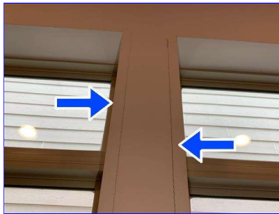
E. Cracking
