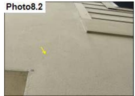
Hairline cracking is present.
