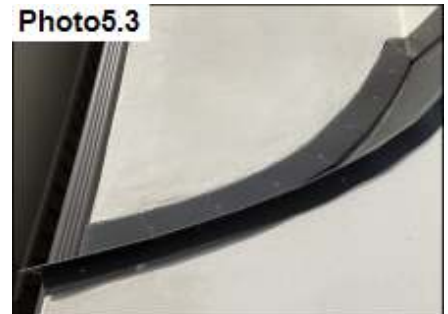
Metal cap is present on top of semi-flat wall.
