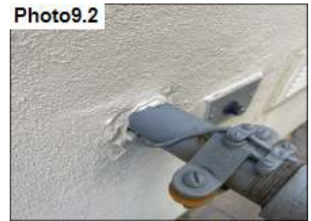
Sealant separation noted around penetrations.
