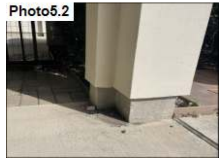
Column base is elevated on a concrete footing.
