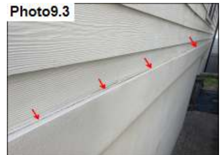
Reverse lap noted at horizontal transition.
