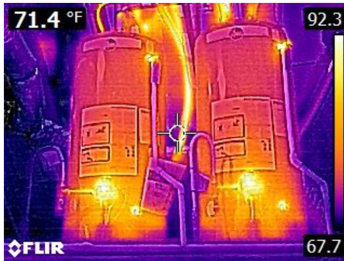
Thermal image of water heater
