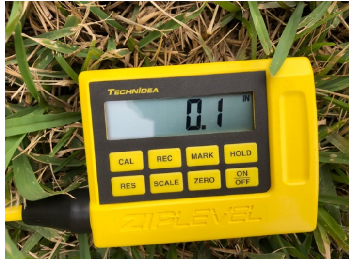
Lot should slope 6" within 10 feet. Grading in this area is flat.
