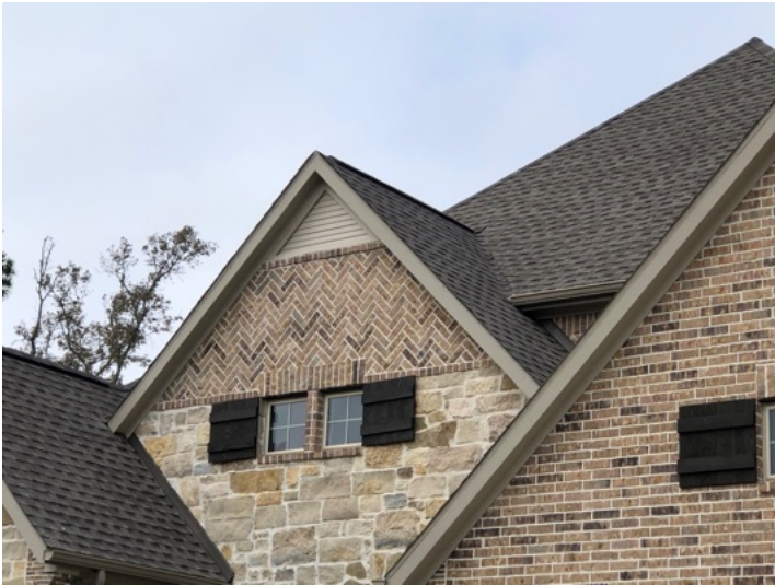
Front roof slope
