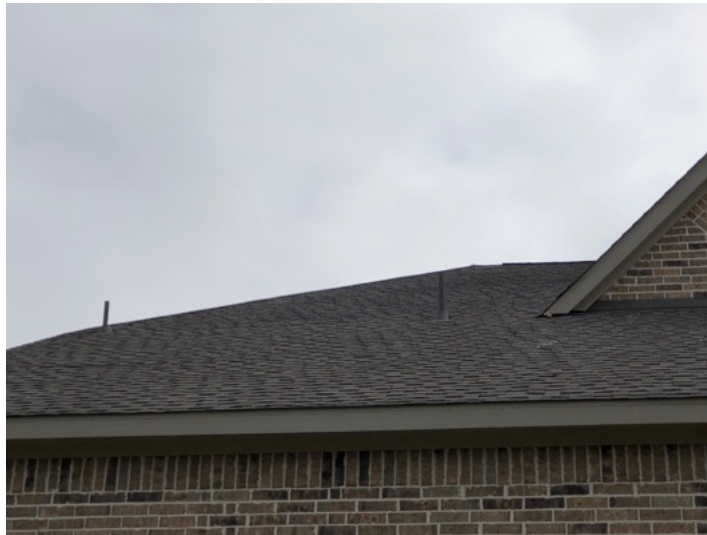
Rear roof slope
