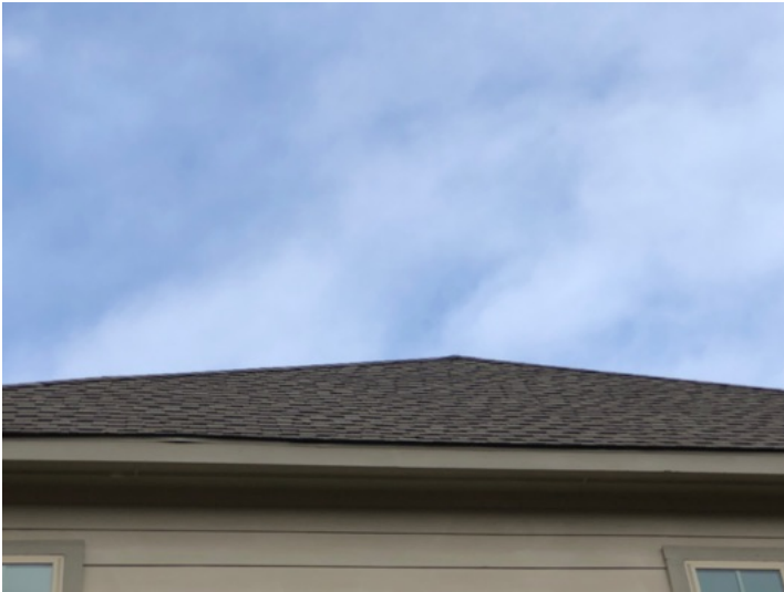
Left side roof slope
