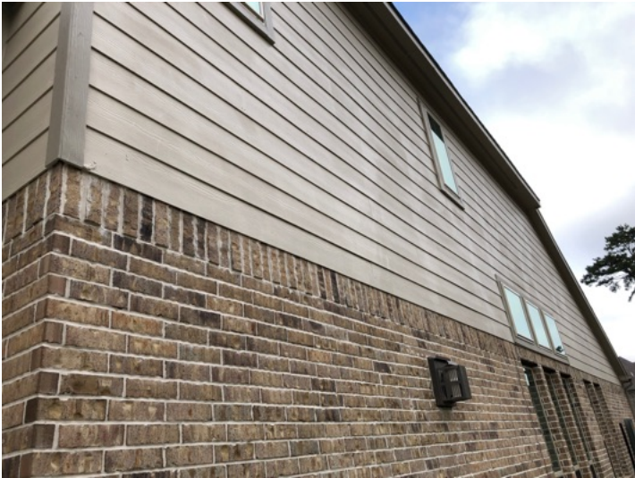
Brick and cement fiber wall cladding
