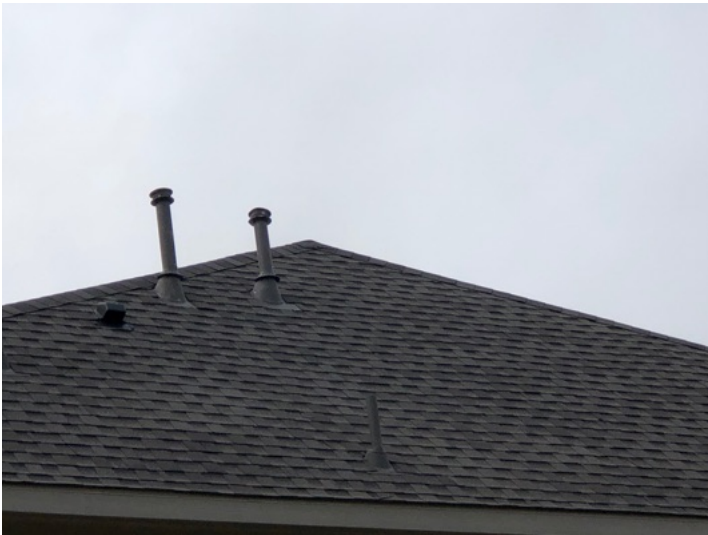
Right side roof slope
