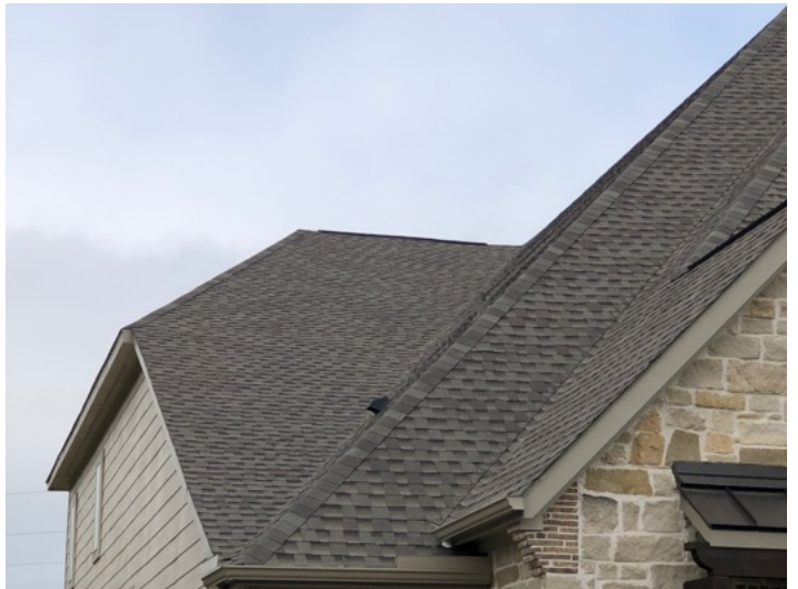
Left side roof slope
