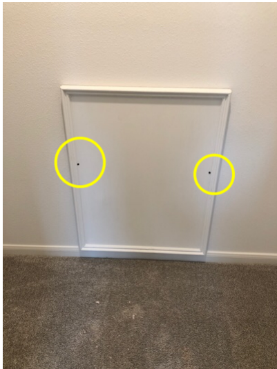
Attic access panel
