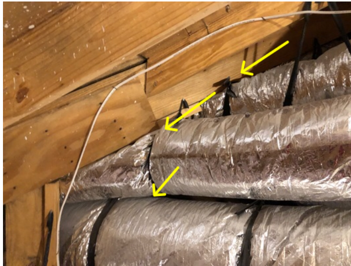
Ductwork compressed
