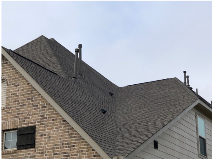
Right side roof slope
