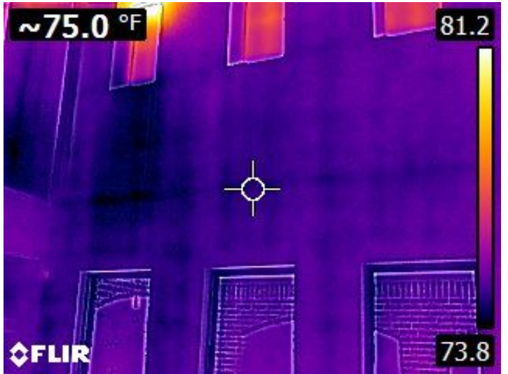
Thermal imaging of walls revealed no significant anomalies
