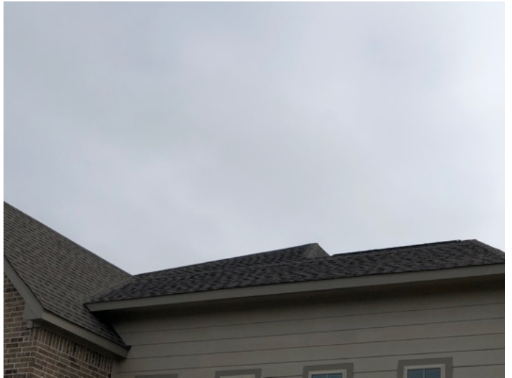
Rear roof slope
