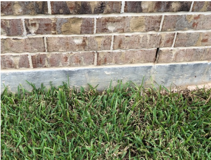
Slab on grade foundation
