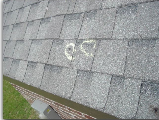
Repair the damaged shingles at the garage roof.
