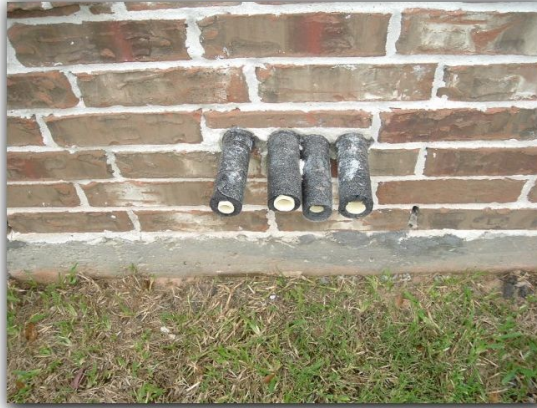
The exterior drain lines need 90 degree elbows installed.
