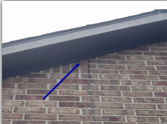
The brick mortar at the left side of the house needs repair.
