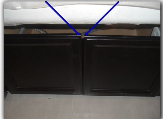
The kitchen sink cabinet doors are out of square and the trim has damage.
