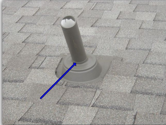
The storm collars at the type B vents require sealant.
