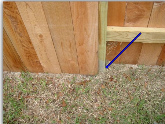
The support posts were not properly set in cement.
