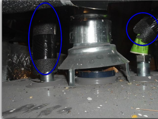
The exterior drain lines need 90 degree elbows installed.
