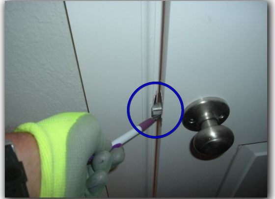
The front right bedroom door latch needs repair.
