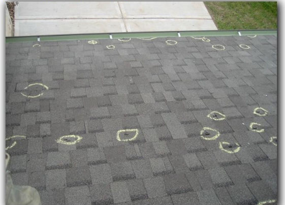
Repair the damaged shingles at the garage roof.
