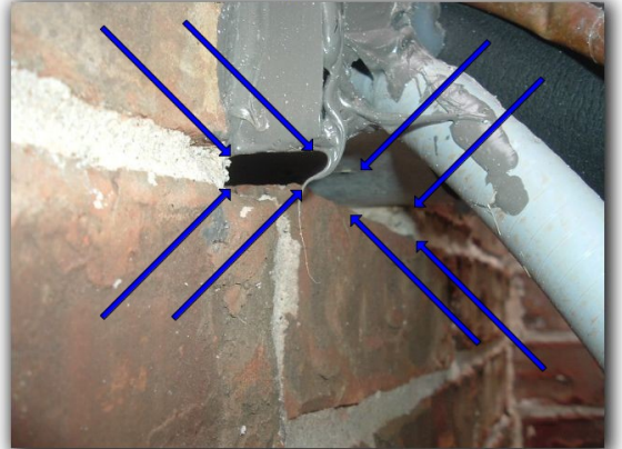
The voids at the exterior freon line needs repair to the sealant.
