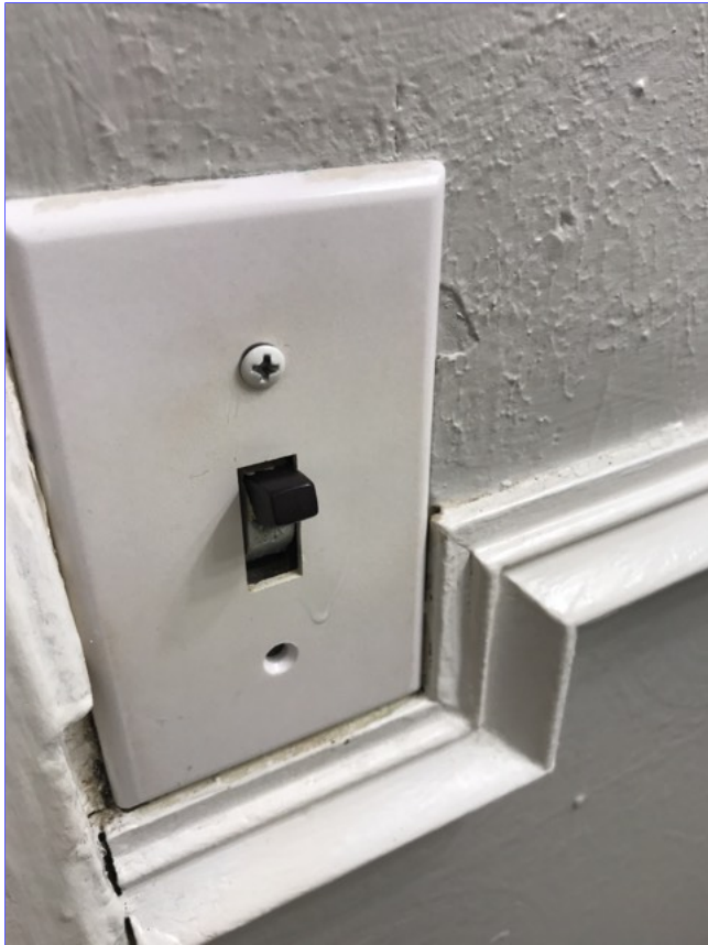
(6) Bedroom and closet walls obstructed by personal belongings. Obstructed areas were not inspected.
