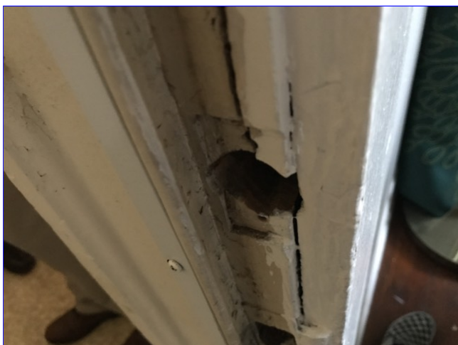
(5) The front entry door is missing a strike plate.
