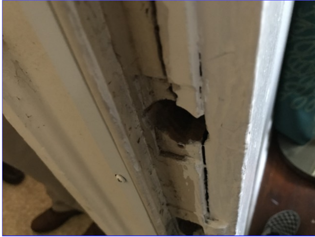
(6) Bathroom closet door hardware does not function.
