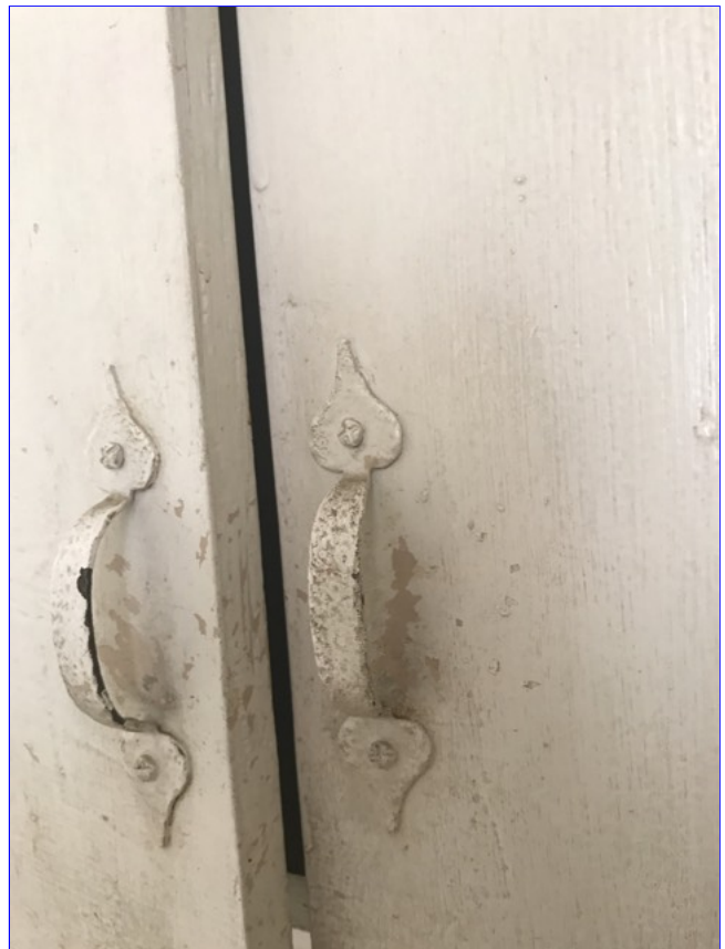
(11) Unit three kitchen cabinets are in poor condition. There are gaps in multiple areas. Doors are non-functioning. Multiple doors do not close.
