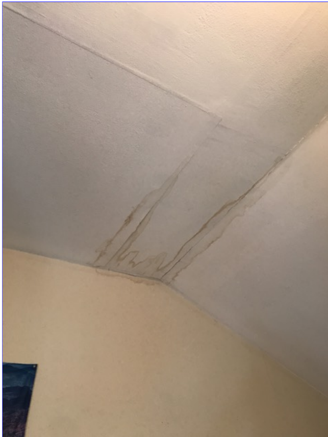
(2) Evidence of moisture intrusion in the ceiling of the bedroom in unit four.
