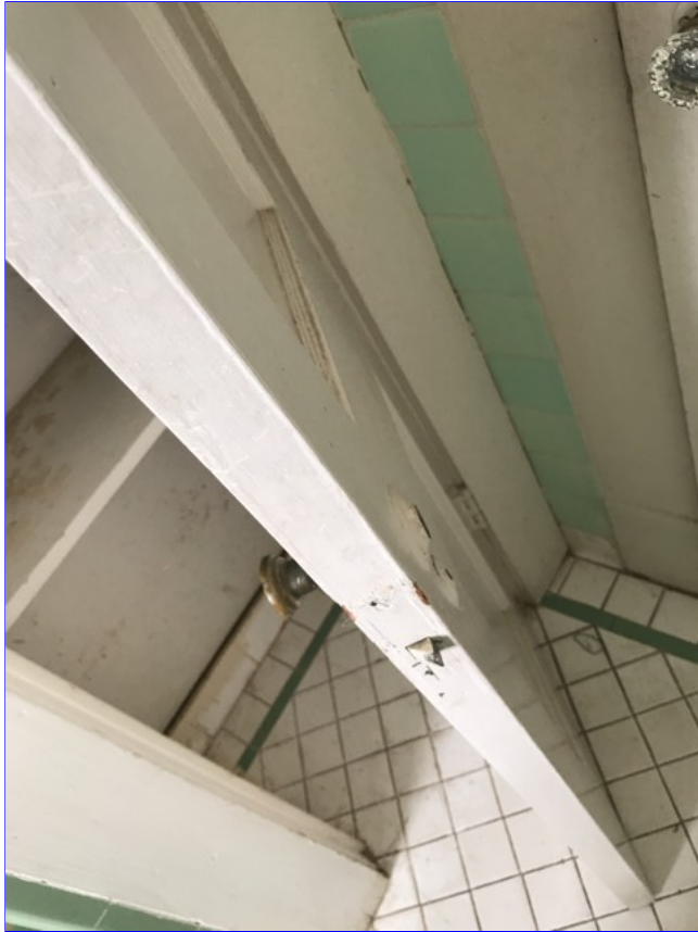
(11) Unit three both entry doors have double deadbolt.
