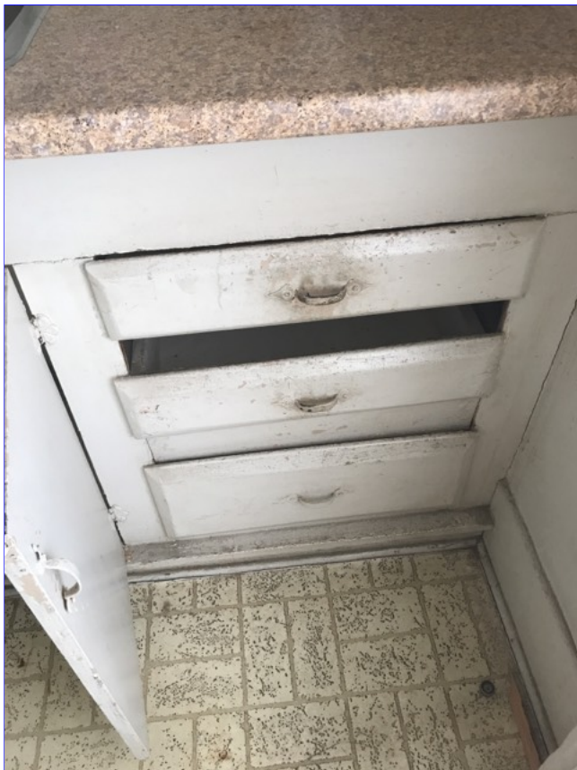
(11) Unit three kitchen cabinets are in poor condition. There are gaps in multiple areas. Doors are non-functioning. Multiple doors do not close.
