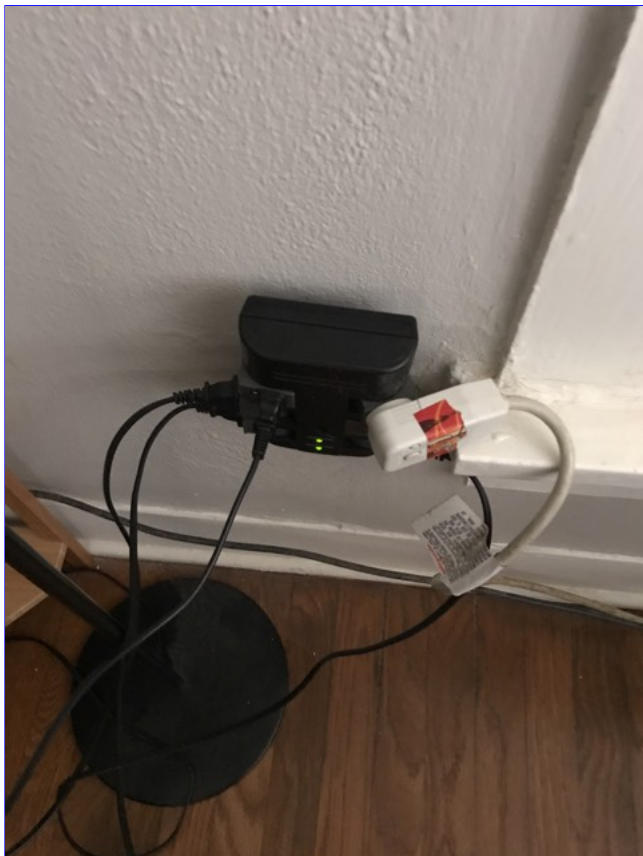
(16) Window air-conditioning unit is plugged into a power distribution center with multiple devices plugged in. The window air-conditioner should have a dedicated 20 amp circuit.
