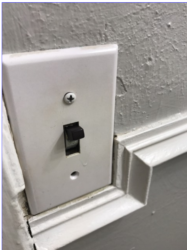
(5) Bathroom light switch plate is missing hardware.
