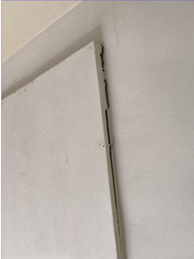
(2) Evidence of moisture intrusion in the ceiling of the bedroom in unit four.
