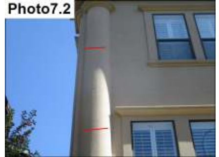
Cracks Noted / Seal & Paint
