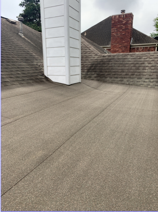
C. Item 5(Picture) The roof covering, is not new and shows signs of wear consistent with its age.
