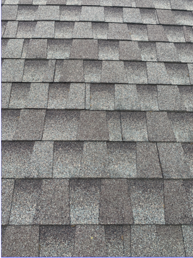
C. Item 1(Picture) The roof covering, is not new and shows signs of wear consistent with its age.
