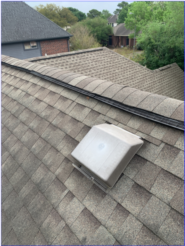
C. Item 6(Picture) The roof covering, is not new and shows signs of wear consistent with its age.
