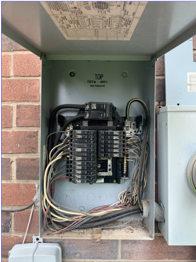
A. Item 1(Picture) The main electrical service panel, shown with dead front cover removed for inspection purposes. The panel inspected okay.
