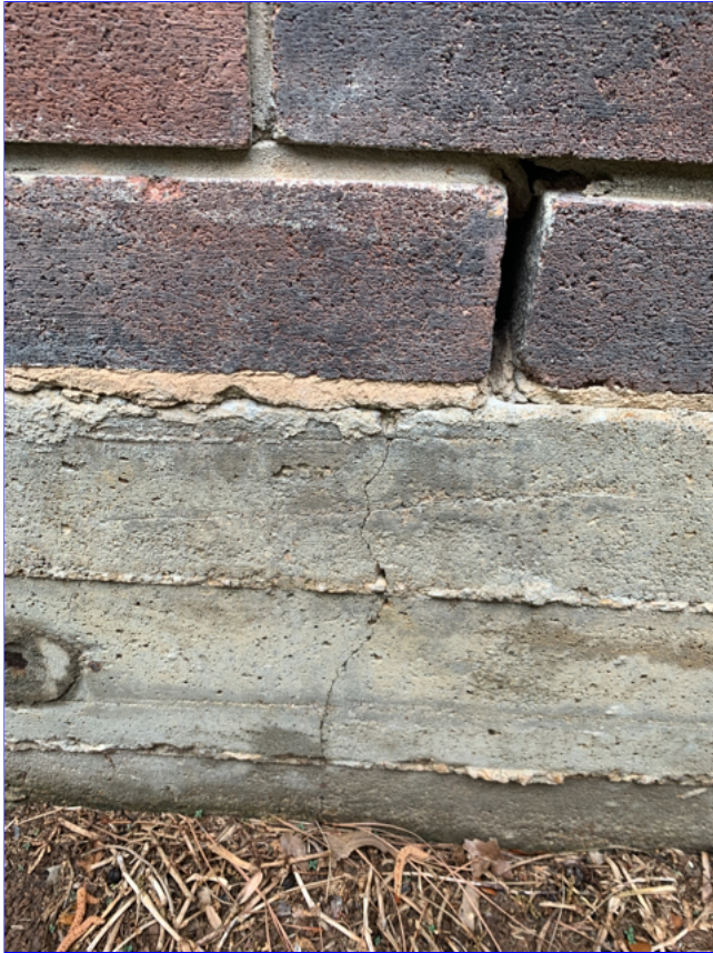
A. Item 3(Picture) There is some slab edge cracking.
