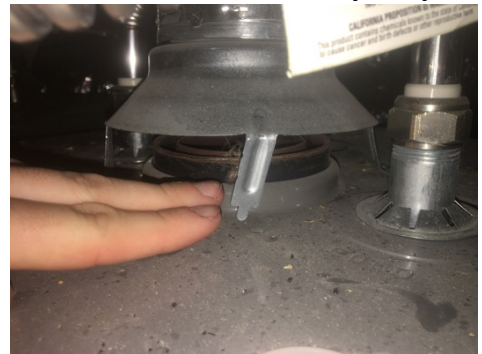
Unit 2: loose diverter leg
