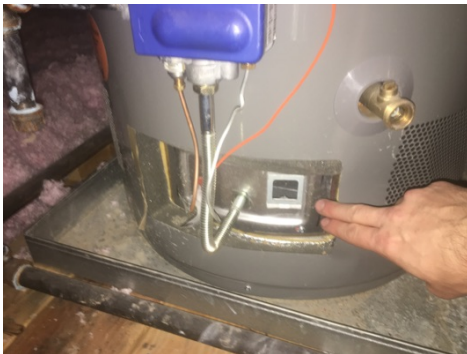
Unit 1: missing shield
