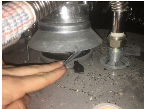
Unit 1: loose diverter leg
