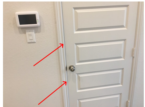
Garage man door: daylight coming through
