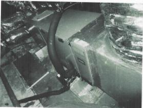
The heating for the house was provided by a electric horizontal furnace located in the attic. The equipment was as follows:
