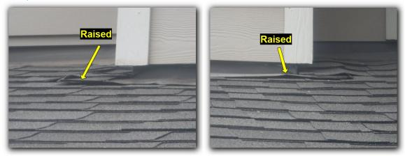
Did not observe kick out flashing installed in one or more areas. Kick out flashing is most important when the siding is made of stucco (this home has brick siding). I have never observed a problem with the lack of kick out flashing on a brick home, but current standards call for kick out flashing to be installed as a preventative measure.
