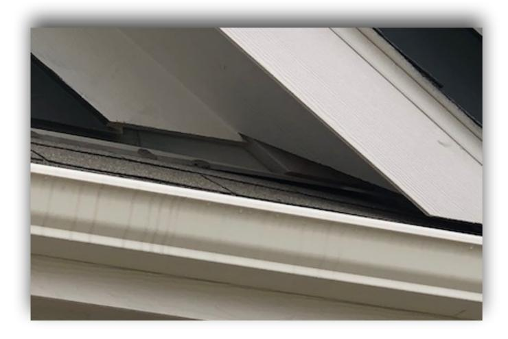
Exterior soffit / fascia eave boards have an excessive gap between roof decking, proper separation is a max of 3/4 inch or less, should be repaired. (over garage)
