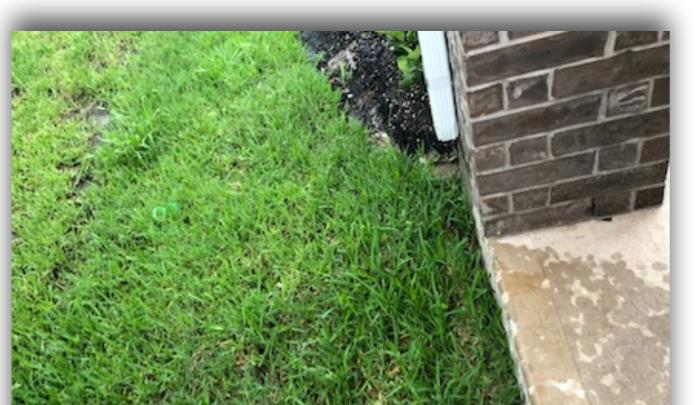
Gutter downspout elbow connection is missing at frontright of home, should be replaced to help divert water away from foundation.
