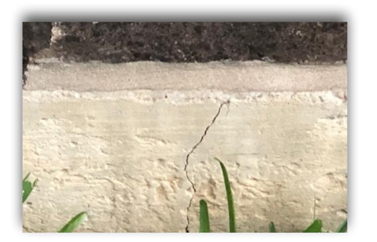
Stress crack(s) noted in foundation slab under right side window - no significant related effects present at time of inspection.
