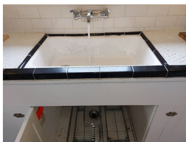
General Photos of Plumbing Fixtures:
