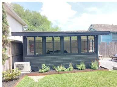
General Photos of Roof Covering:
