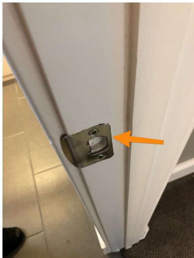
Strike plate needs an adjustment.
