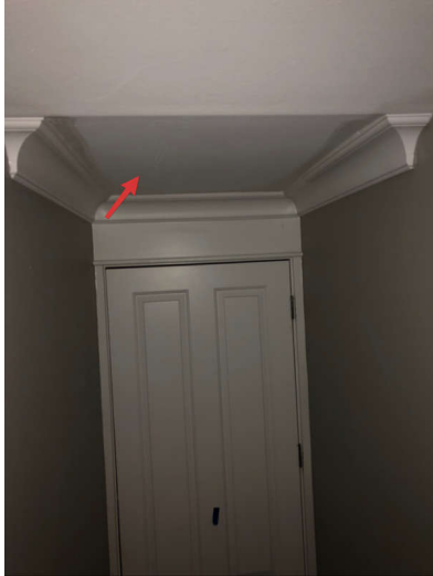
Garage apt entrance
