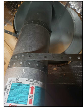
Roof vent penetration
