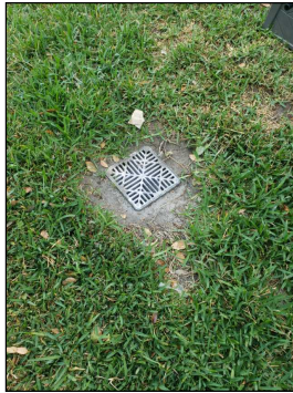
Drainage system noted
