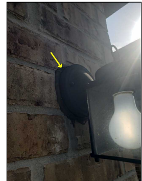
Front, reseal around outdoor light fixture
