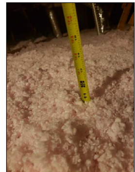
Insulation is 10 to 11 inches deep
