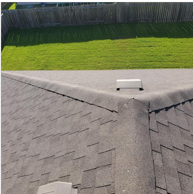
C. Item 4(Picture) Roof overview
