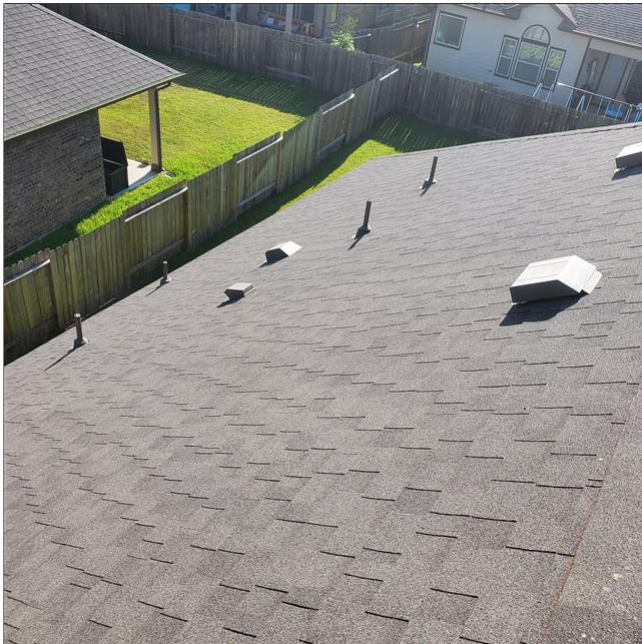
C. Item 2(Picture) Roof overview
