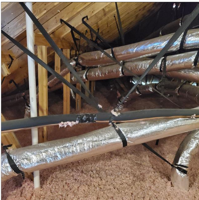
D. Item 1(Picture) Attic overview.
