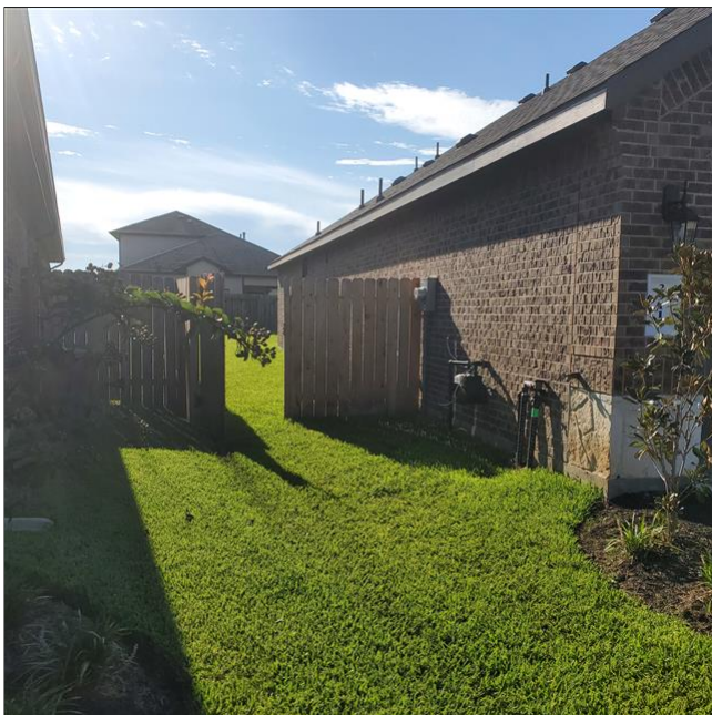
B. Item 1(Picture) Ground properly sloped away from the home.
