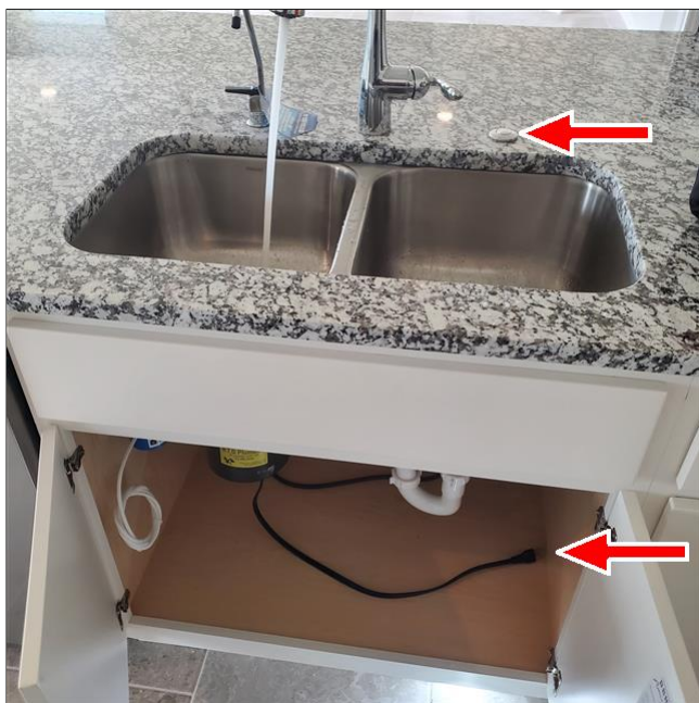
B. Item 1(Picture) Button did not shut disposal off. Unit had to be unplugged.
