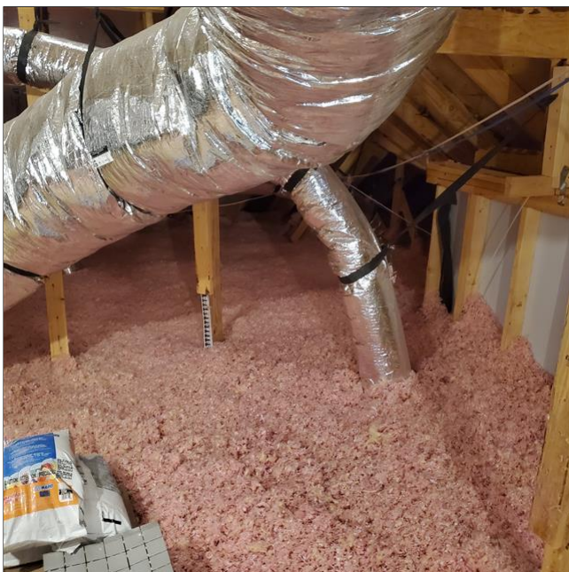
D. Item 2(Picture) Attic overview.
