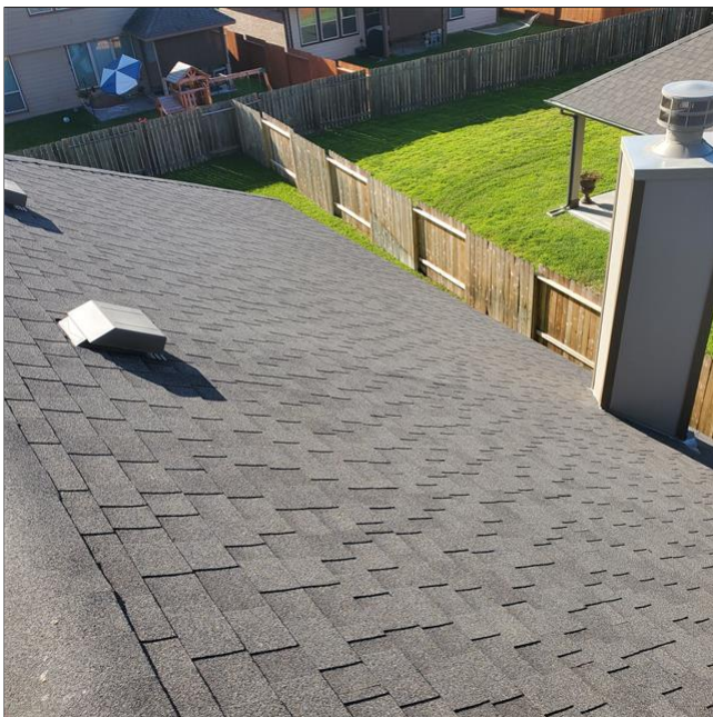
C. Item 3(Picture) Roof overview
