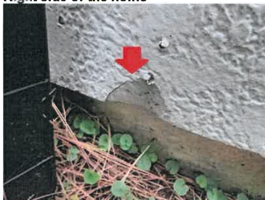
Seal up siding/bricks around the home to prevent moisture penetration: Both sides of the garage door
