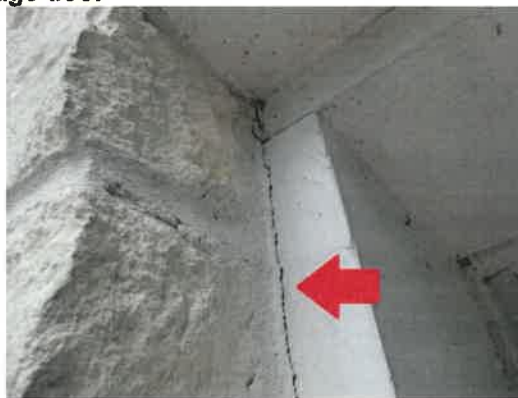
Seal up siding/bricks around the home to prevent moisture penetration: Both sides of the garage door
