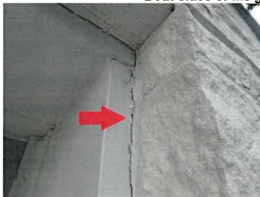
Seal up siding/bricks around the home to prevent moisture penetration: Both sides of the garage door
