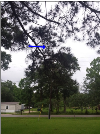
-Electrical feeds were running through the trees, recommend trimming limbs from wires.
