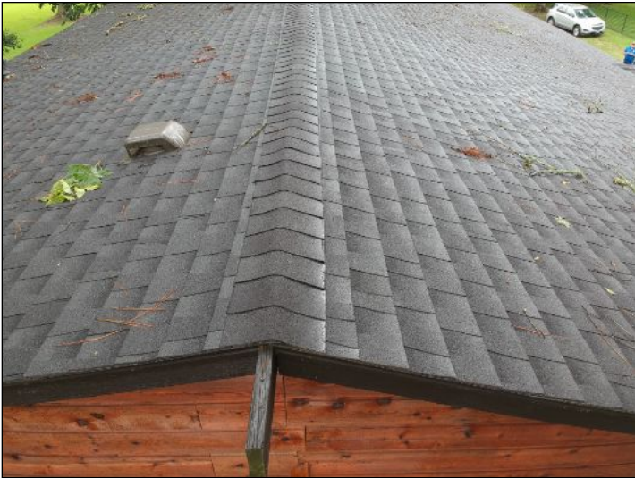
Overview of roof
