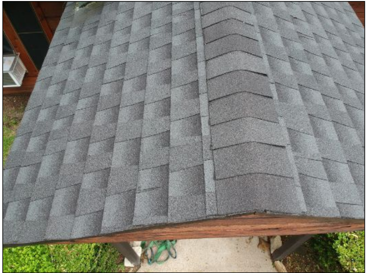
Overview of roof
