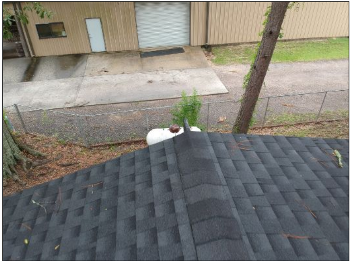
Overview of roof
