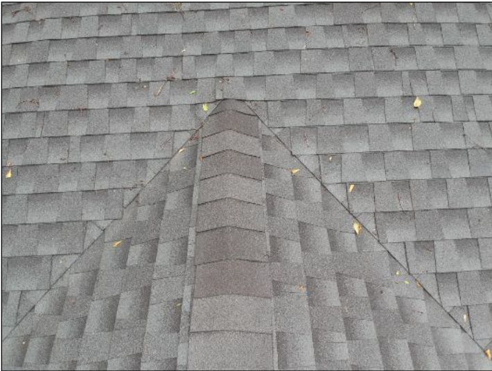
Overview of roof
