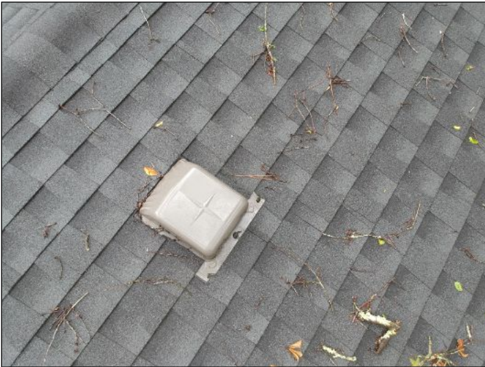
Overview of roof
