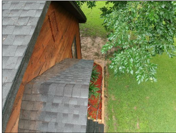
Overview of roof
