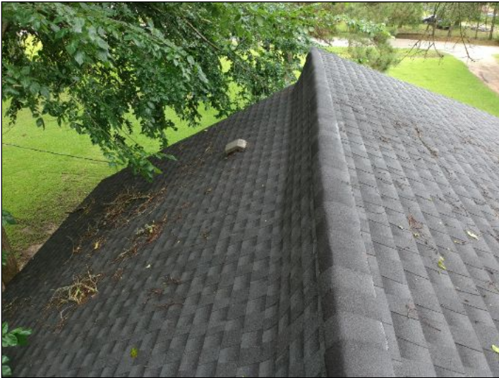
Overview of roof
