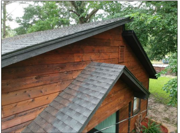
Overview of roof
