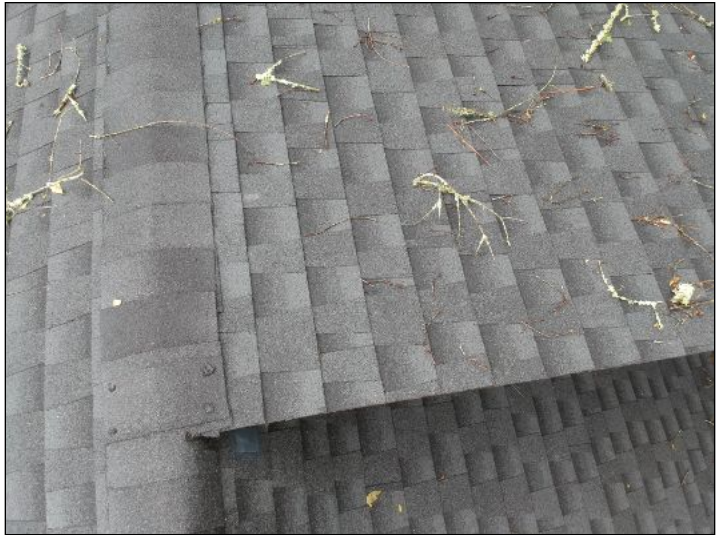
Overview of roof
