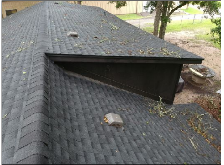
Overview of roof
