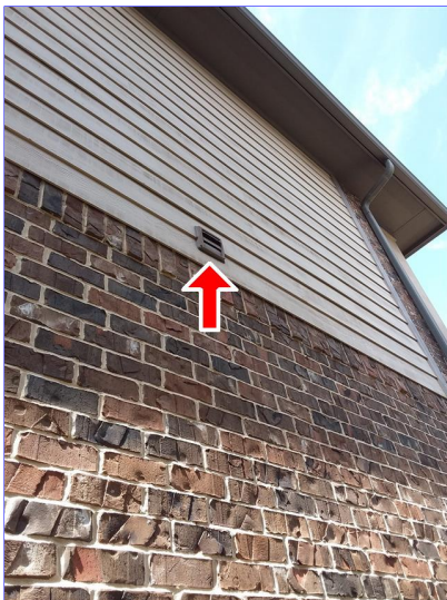
F. Item 2(Picture) left
