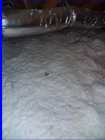
blown insulation 14 inches
