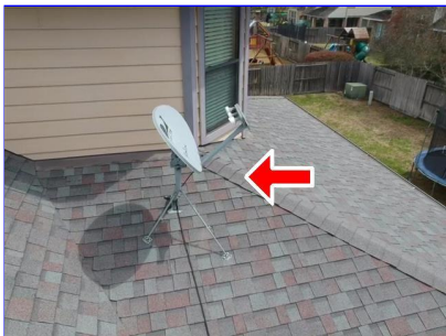
C. Item 1(Picture) rear right
