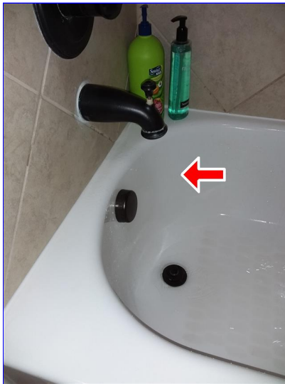
A. Item 1(Picture) shared bath
