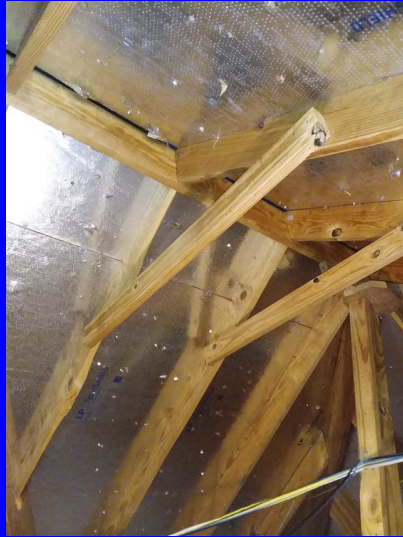
stick built roof structure w/radiant barrier
