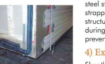
steel straps. This multiple-step strapping process keeps the structure of the home intact during strong winds, helping to prevent leakage.
