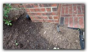
Patio is too high on the wall. Cannot inspect foundation and is considered a conducive condition to wood destroying insects.
