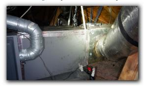
Observed several / multiple areas in attic where flex duct touch and are missing required
