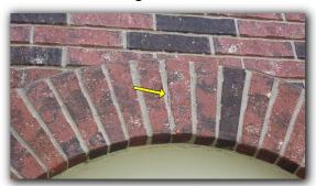
Cracks in brick arch observed, loose bricks are hazardous.
