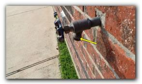
Gas piping not sleeved as it passes through masonry wall as required by Code [CABO 2608.3] IRC 2603.3.
