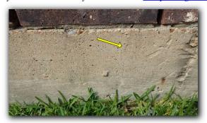
Spalling at one or more locations around house / garage. Generally due to not enough concrete (Minimum 2") coverage over steel in foundation which causes steel to rust and spall / pop off concrete.
