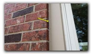
Window brick ledge should have a positive slope to shed water. The slope should be a minimum 15 degrees.
