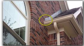
One or more areas of raised shingle tabs from fasteners not secured down properly or nail heads popping up through shingles.
