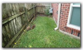
Buyer's note; inspector observed flower bed / soil has been trenched around some areas of house/garage. It is our experience that the soil soon fills up the trench resulting in soil at/above/in contact with house siding and foundation resulting in wood rot and/or water entry during heavy rains.
