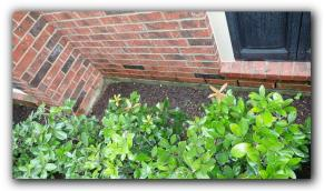
Ants entering house at masonry weep holes, use insecticide treatment, do not seal up weep holes.
