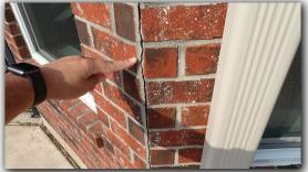
Caulking missing and/or deficient around trim boards may allow wind driven rain entry.
