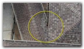
Rusted flashing can be a potential location of wind driven rain entry.
