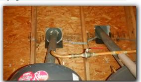
The vent hood is not properly aligned with the vent pipe. This condition allows dangerous combustible gases to enter the structure instead of properly venting to the exterior.
