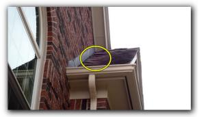
Lower side of flashing is not sealed down, wind driven rains can cause water penetration.
