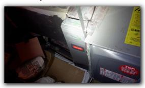
Some staining and possible mold on plenum box/joints. Recommend cleaning.
