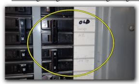
Dead front was painted to the wall and was not removed for inspection because removing the cover may damage the wall finish.
