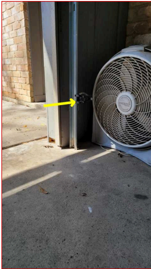
The garage door sensors should be installed within {6"} of the finished floor.
