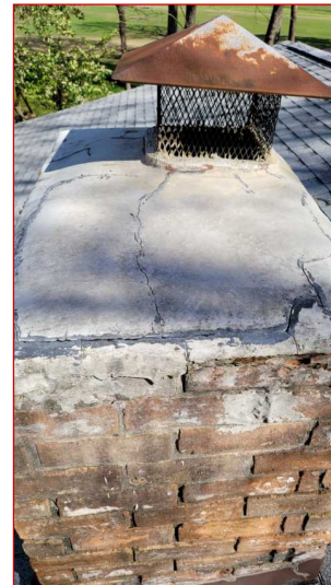
Mortar cracked.
