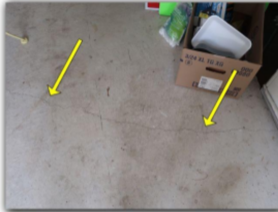
Cracks in exposed concrete floors
