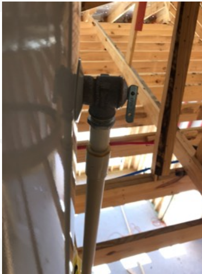
Temperature pressure relief valve
