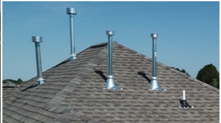
Roof Covering Materials
