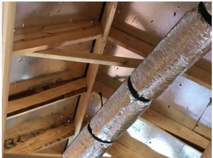
Roof Structures and Attic space
