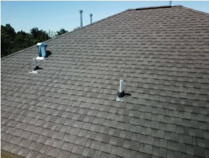
Roof Covering Materials
