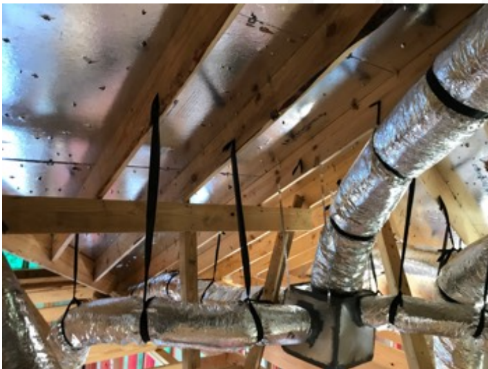
Roof Structures and Attic space
