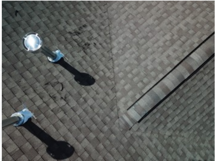
Roof Covering Materials
