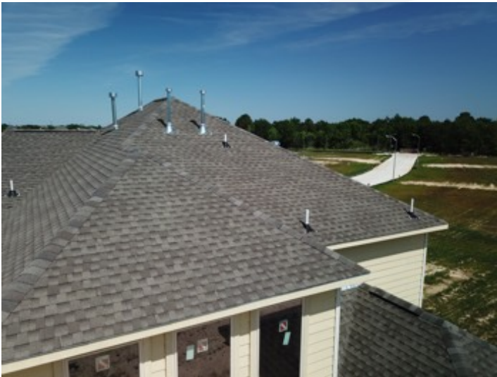
Roof Covering Materials
