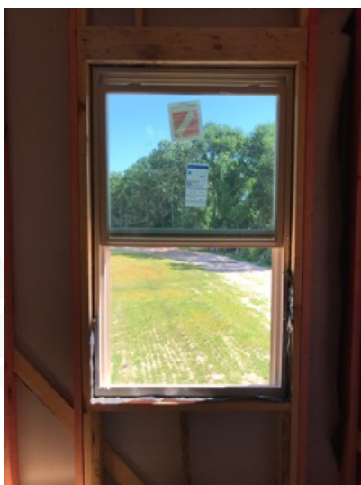
All windows are functional
