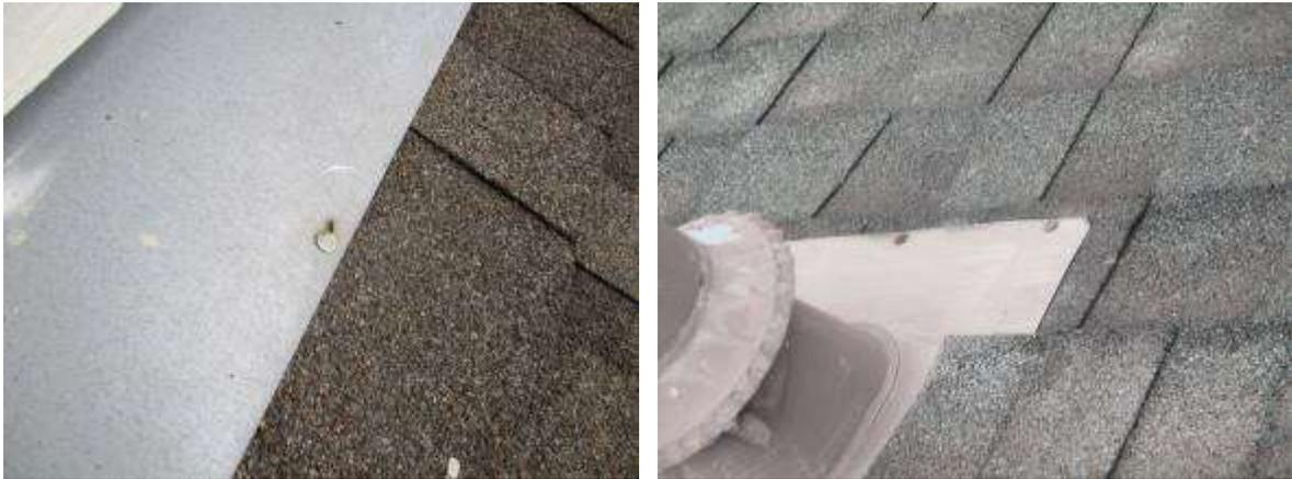
We observed rust on some of the metal roof accessories, and although the accessories are still performing their intended function, it is recommended that the rust be removed. Locations included: Metal valleys
