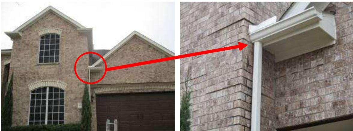
The downspout was missing a splash block.
